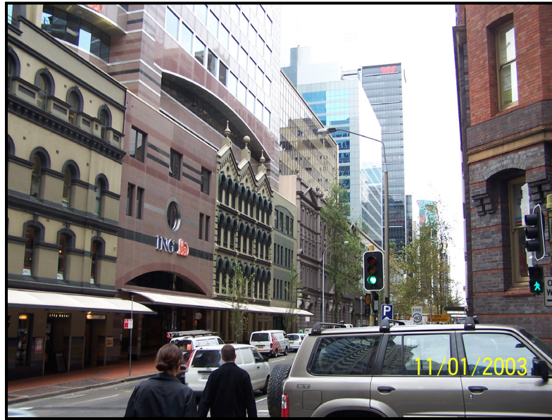
Figure 6: West side of Kent Street, opposite the site, illustrating existing street wall and setbacks.
