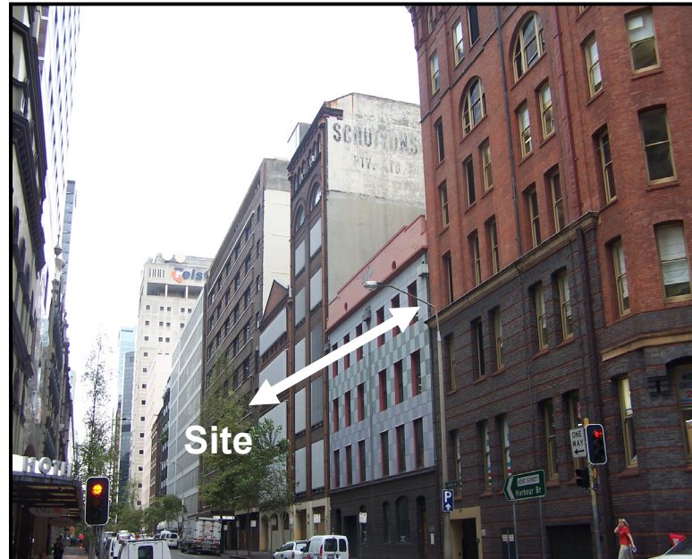
Figure 2: Kent Street view of the site looking North
