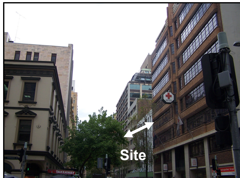
Figure 3: Clarence Street view of the site looking South
