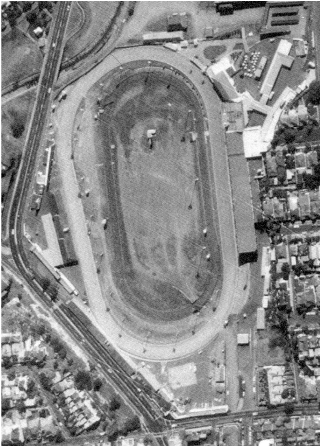
Figure 2.7: 1982 Aerial Photo. Lands Department Aerial Photograph Sydney 1982 Run 22 NSW 4241-141
