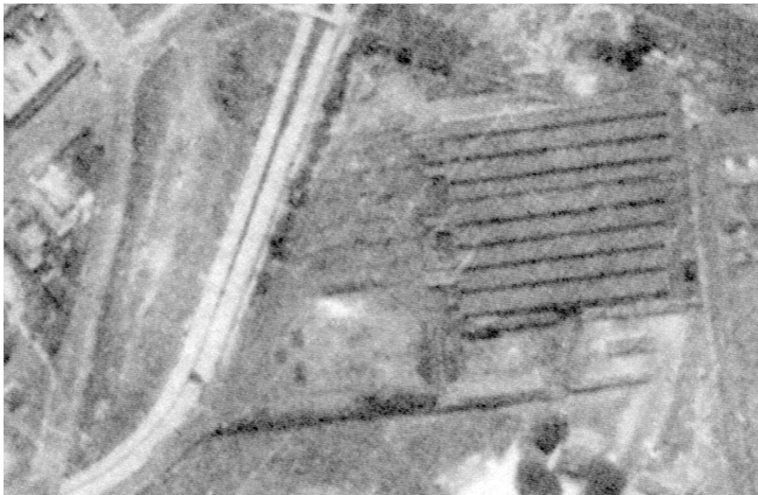
Figure 2.13: Aerial photo, March 1930. Lands Department Aerial Photograph Map 3422 Sydney Run
