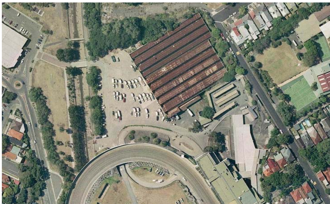
Figure 2.18: 2009 aerial photo of the Tramsheds precinct. NSW Lands Dept Six Viewer.
