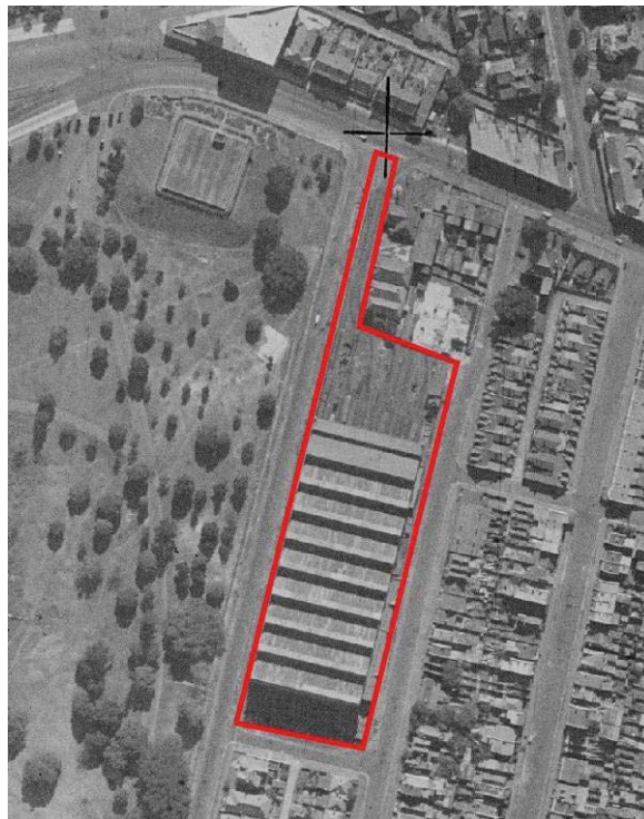
Figure 4.35: The layout and park side setting of Waverley Depot in 1943. Source: NSW Roads and Traffic Authority, 'From the skies' CD-ROM
