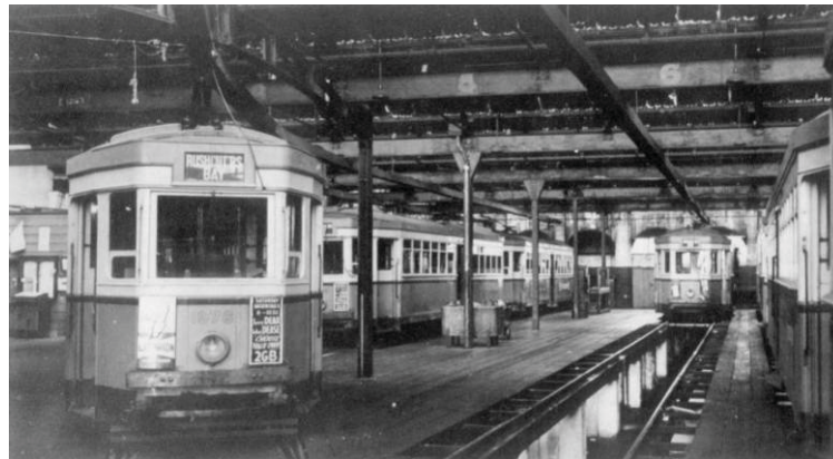
Figure 4.57: The interior of the shed at Rushcutters Bay at the time of its closure. Source: Keenan, David, The Watson's Bay Line of the Sydney Tramway System , Transit Press, Sans Souci, 1990, p.82
