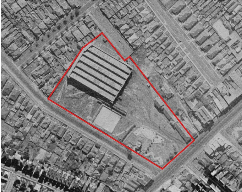
Figure 4.50: The configuration and suburban setting of Tempe Depot in 1943. Source: NSW Roads and Traffic Authority, 'From the skies' CD-ROM
