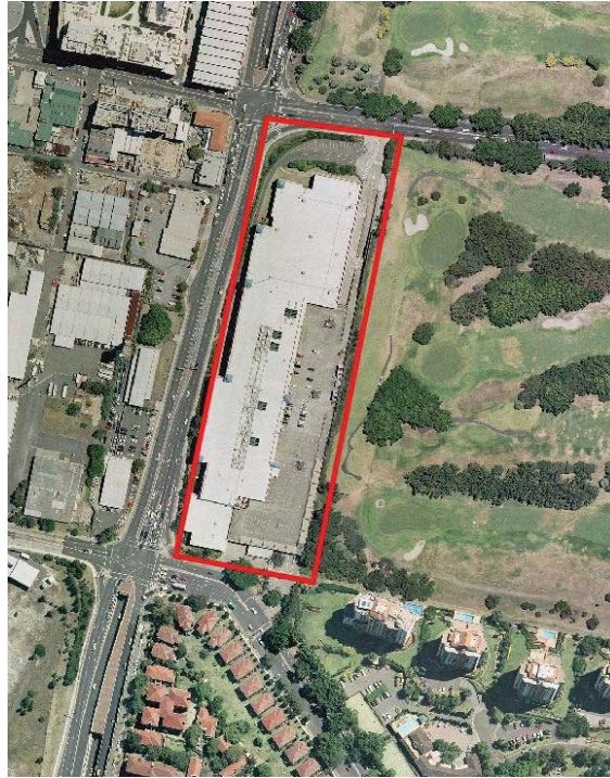
Figure 4.48: The redeveloped site of the former Dowling St depot today. Source: NSW Lands Dept Sixviewer
