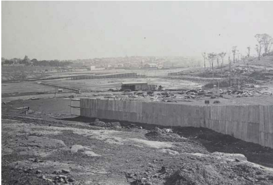
Figure 6.4 A record of the work being undertaken on 6 th April 1899 in reconstructing the Lillie Bridge Recreation Ground into the grounds of the Forest Lodge Racing Club. Looking north from Wigram Street to Rozelle Bay showing the denuded and reclaimed floor of the shallow valley of Allen's Bush. The iron fence depicted is a remnant of the original Lillie Bridge Ground.
