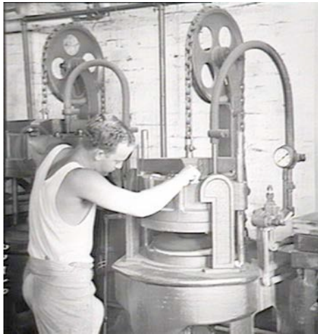
Figure 5.3.2 Rolling the brim with steam under great pressure
