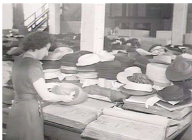
Figure 3.2 Quality control and checking. Both the staircase and hardwood columns are visible. March 1949
