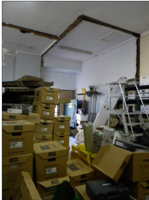
Figure 74: Evidence of removed partition walls. Figure 75: Openings with metal caging.
