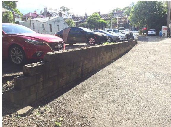
Figure 40: View of the sandstone retaining wall for the access road to the south of the warehouse building
