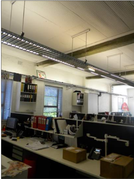
Figures 54 and 55: First floor interiors, showing partitioning and exposed bearers with corrugated steel lined ceilings.
