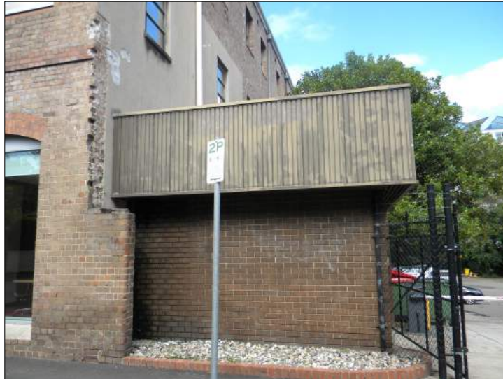
Figure 45: Evidence of alteration to the eastern elevation. The moulded corner bricks suggest an opening in the removed wall.
