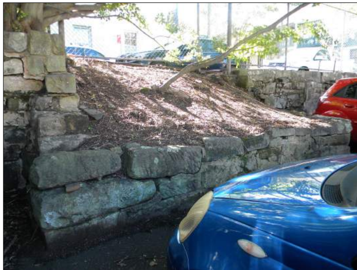
Figure 40: Section of the sandstone retaining wall along the eastern (Junction Street) boundary.
