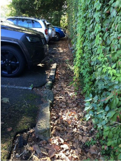
Figure 49: View of the sandstone drain that is aligned to the southern extent of the property, providing drainage from Junction Street towards Orphan School Creek
