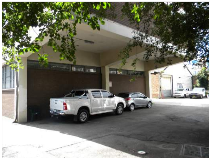
Figure 66: The cantilever on the western side.
