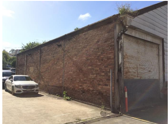
Figure 38: View of the brick retaining wall between the northern carpark and the warehouse building
