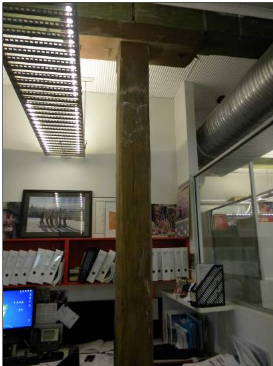
Figures 54 and 55: First floor interiors, showing partitioning and exposed bearers with corrugated steel lined ceilings.
