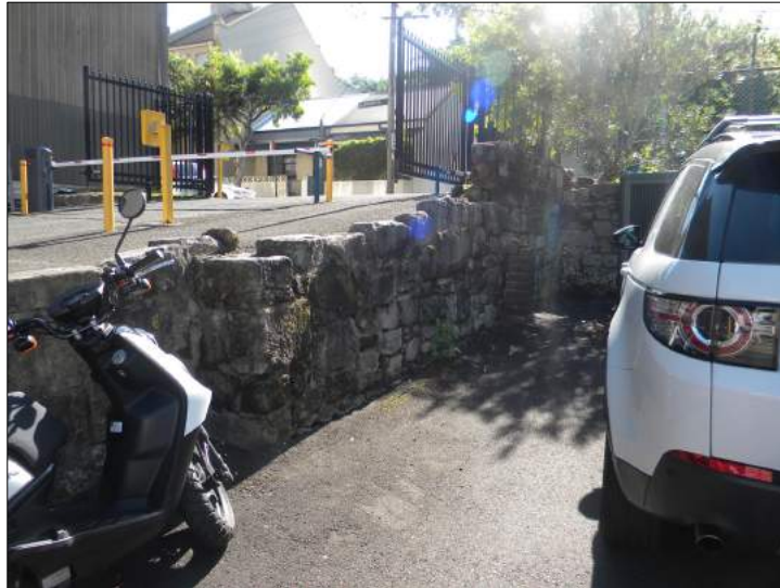
Figure 39: The southern-most entrance off Junction Street, showing the sandstone retaining wall that allows for the fall in the site. Also showing the northern most extent of the stone wall along the eastern boundary.
