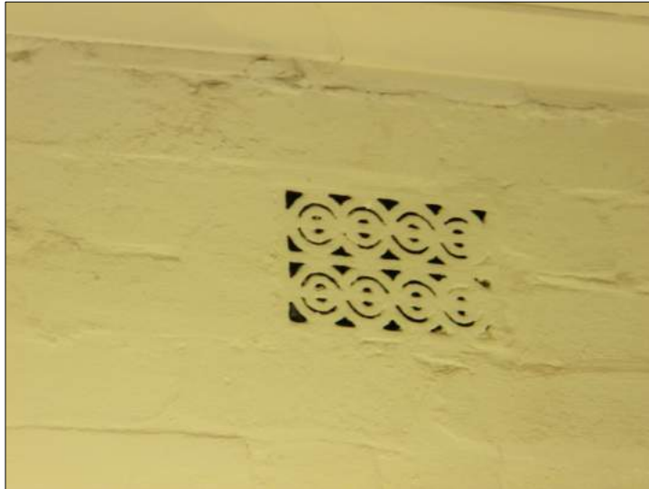
Figure 57: Detail of a wall vent set in the exterior wall.
