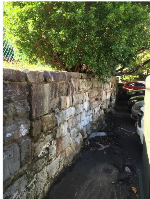
Figure 44: View of sandstone retaining wall between Junction Street (at a higher level) and the southern carpark (lower level)
