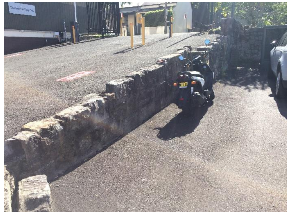
Figure 40: View of the sandstone retaining wall for the access road to the south of the warehouse building
