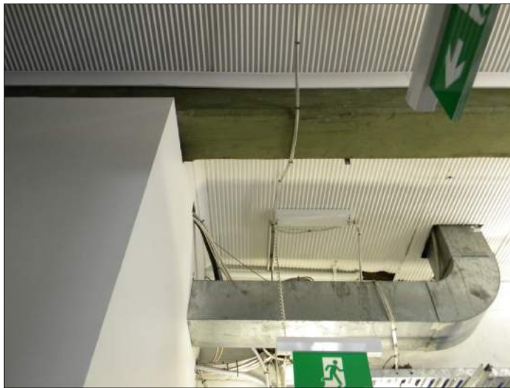
Figure 58: Detail of the corrugated metal sheet ceiling with simple cornice detail against the beam.
