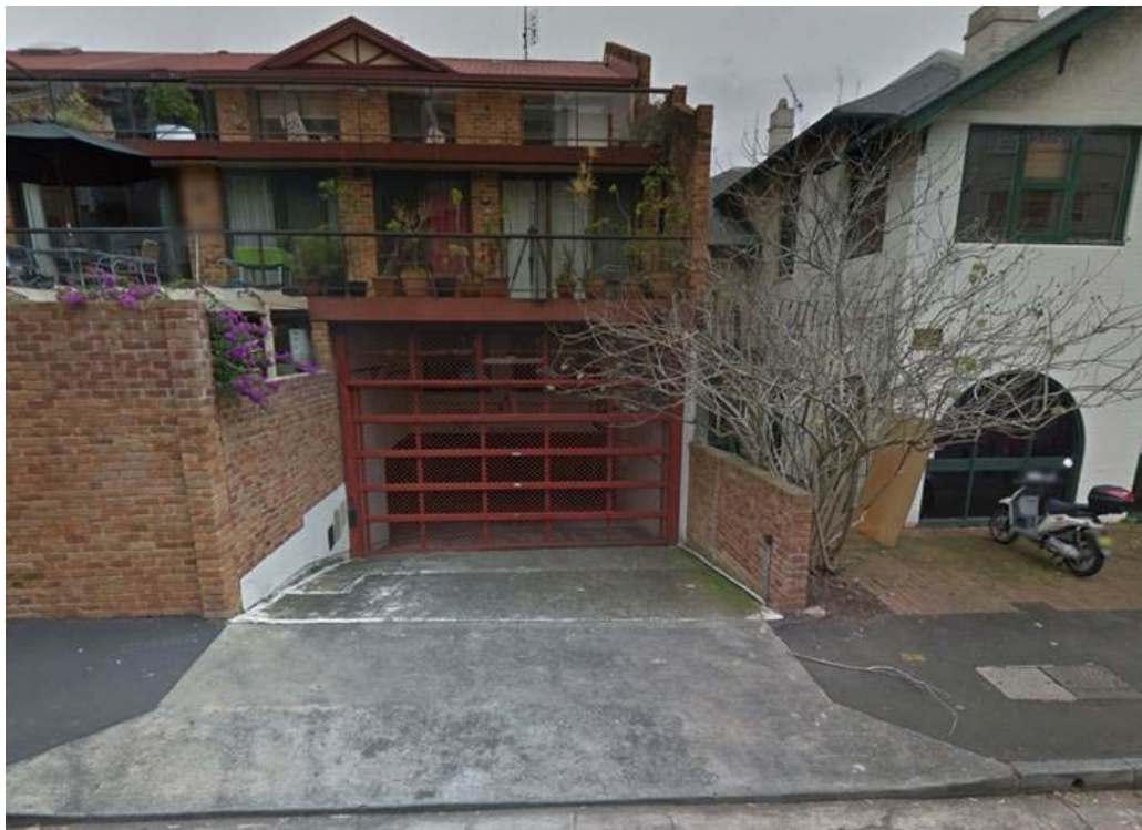
Figure 4: Front external view of boundary condition, shutter and overhang above driveway
