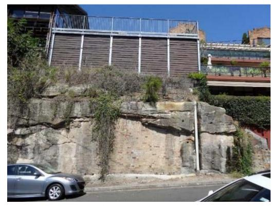
Figure 32: View of brick infill in existing cliff face
