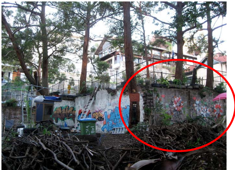
Figure 4: Image of Wall in approximately 2009
