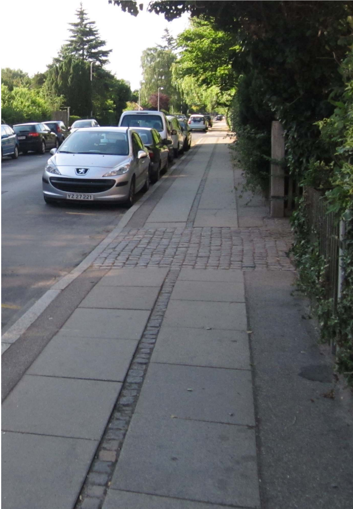
Example 3 – a contrasting, recessed cobble is used in conjunction with pavers for directional travel
