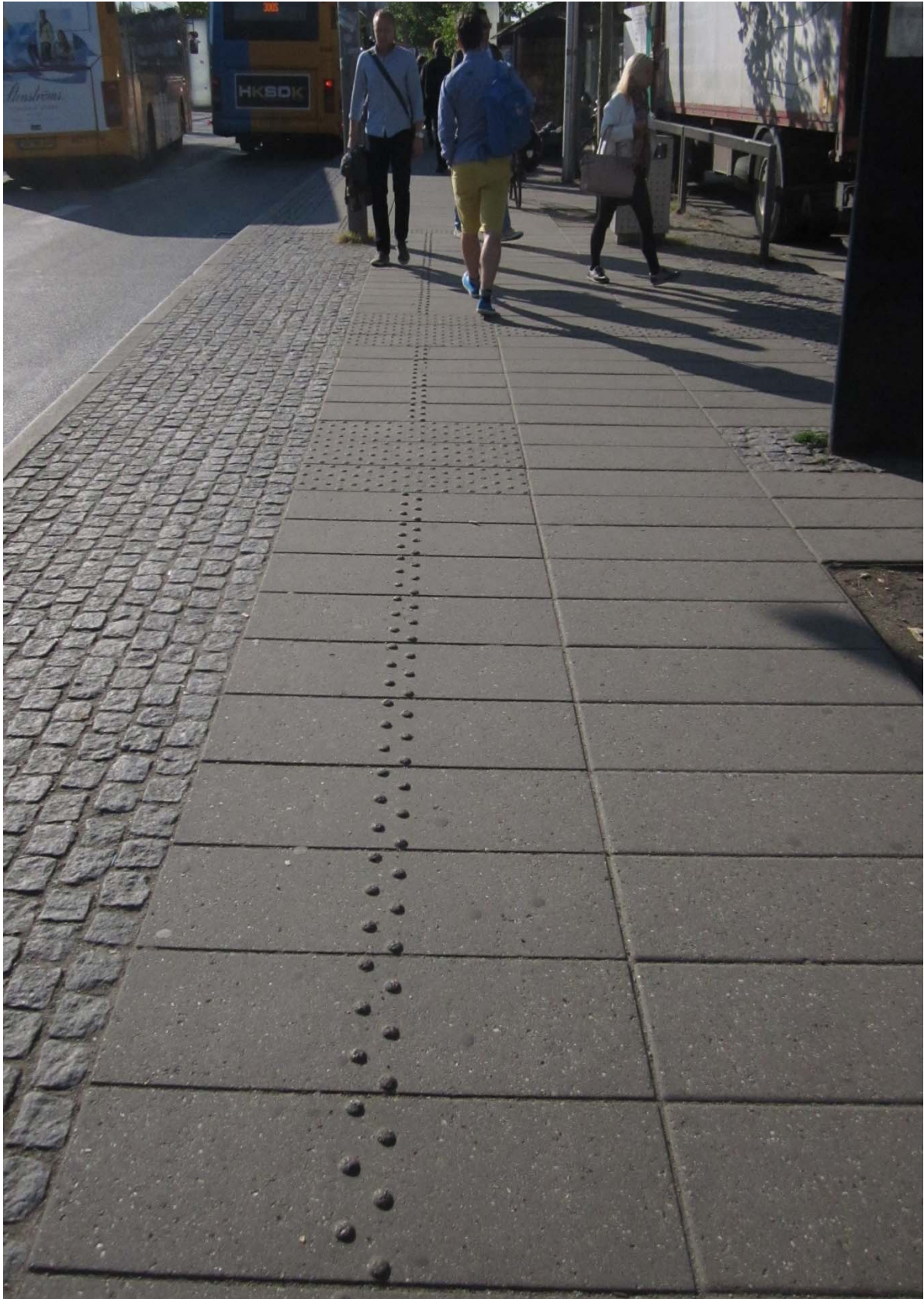
Example 2 – paver with discrete, texturally contrasting raised dots for directional travel.
