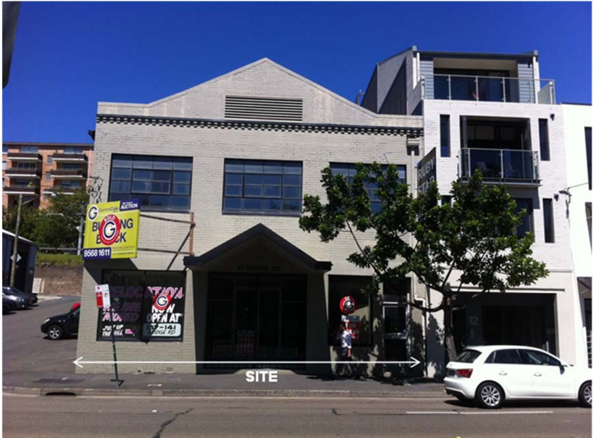
Figure 3: Bridge Road (north-western) elevation.
