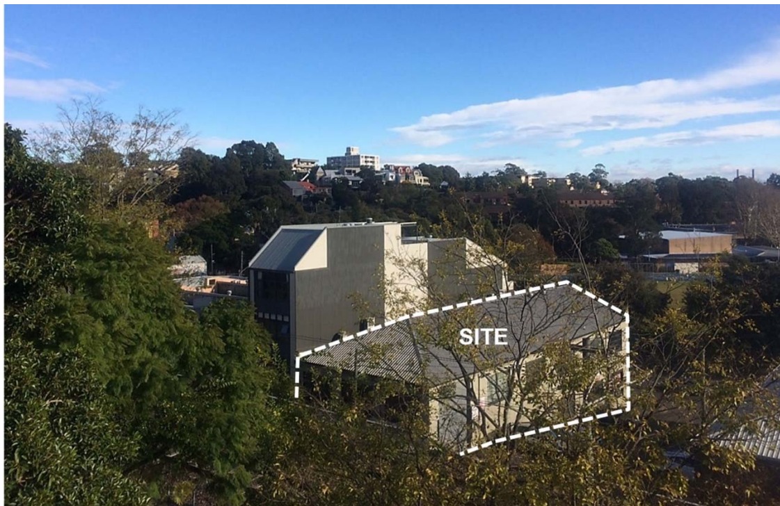
Figure 23: View from Darghan Street level car park of Blackwattle apartments.
