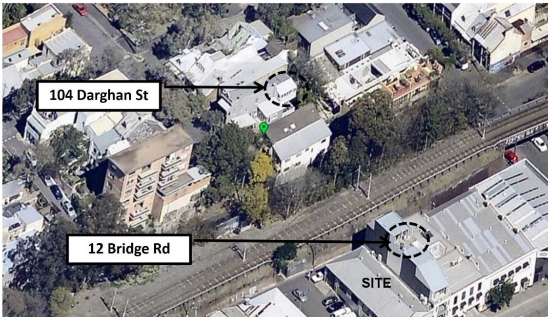
Figure 25: North-facing balcony adjoining bedroom of 104 Darghan Street and level 5 balcony of 12 Bridge Road circled in dashed black line.
