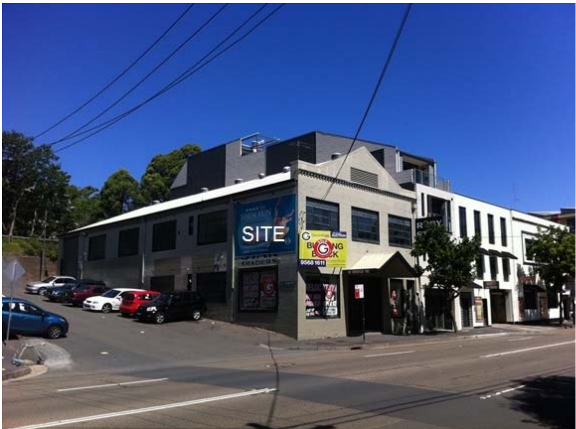
Figure 2: Subject site on the corner of Darghan Street and Bridge Road.
