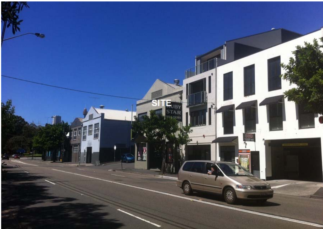
Figure 6: Looking north-east along Bridge Road.
