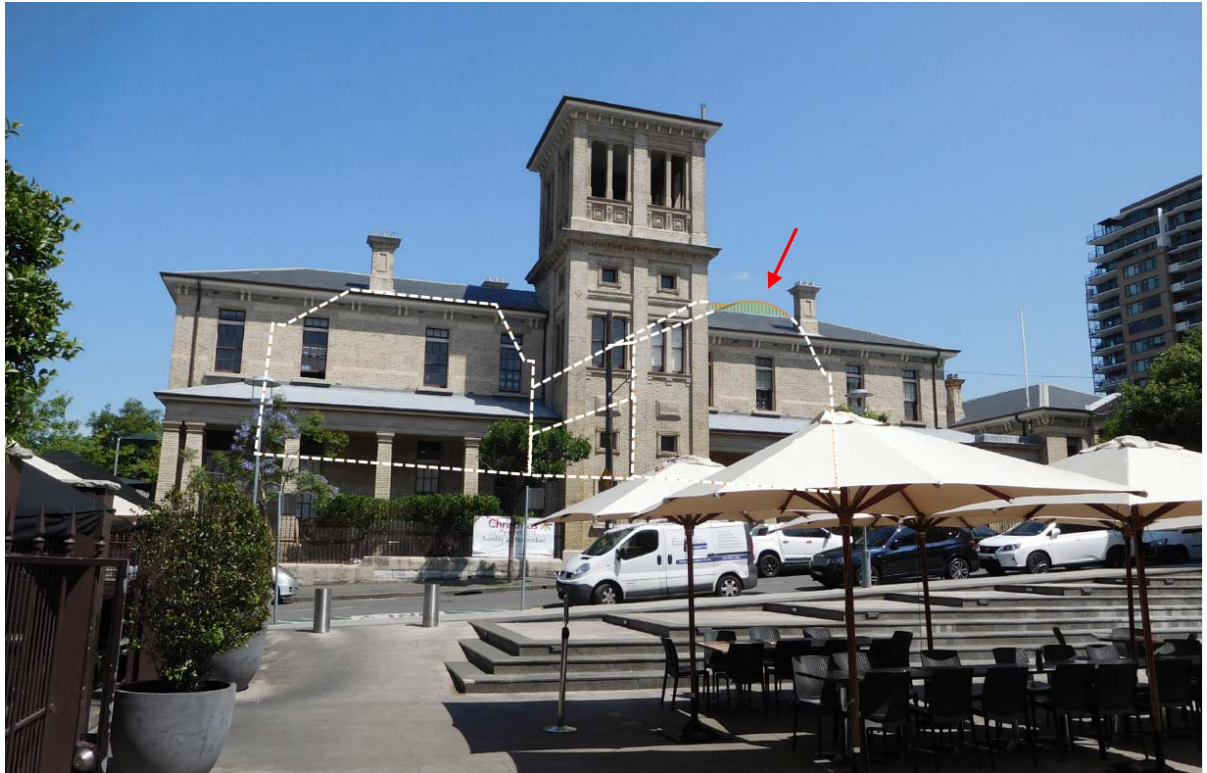
Figure 1 – View from John Street Square (with unseen building envelope shown in white dashed line). The only visible element is the receding roof of the Mount Street terrace (identified by arrow).
