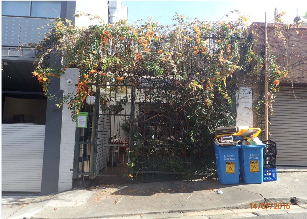
Photograph 1: Existing rear fence at subject site, as viewed from Nimrod Street.
