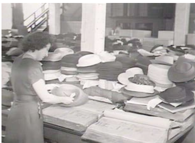
Figure 5.3.8 Quality control and checking. Both the staircase and hardwood columns are visible. March 1949
