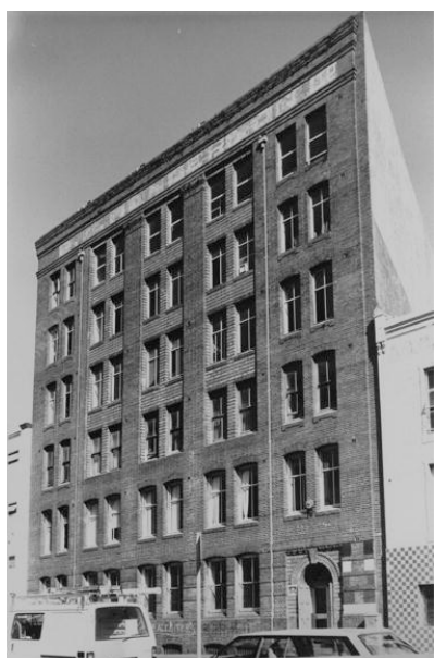
Figure 5.3.10 Former Henderson factory in 1978
