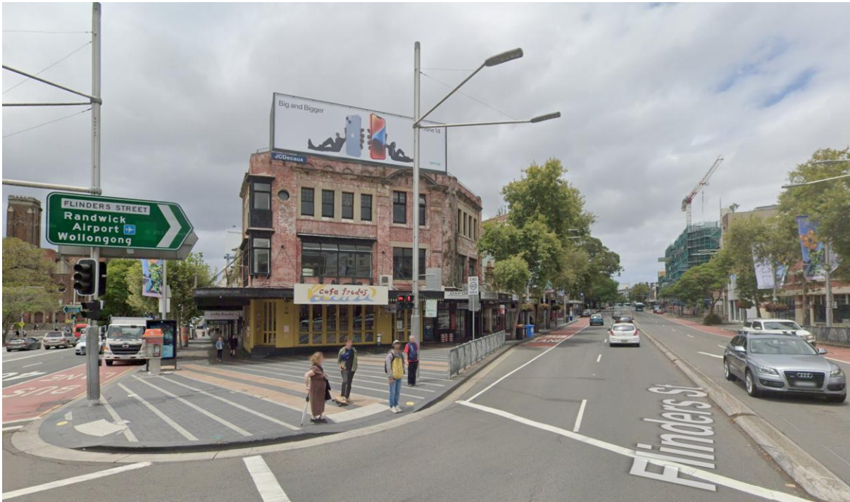
Figure 5 – View of existing roof advertising sign on 195 Oxford Steet (Source: Google Maps).
