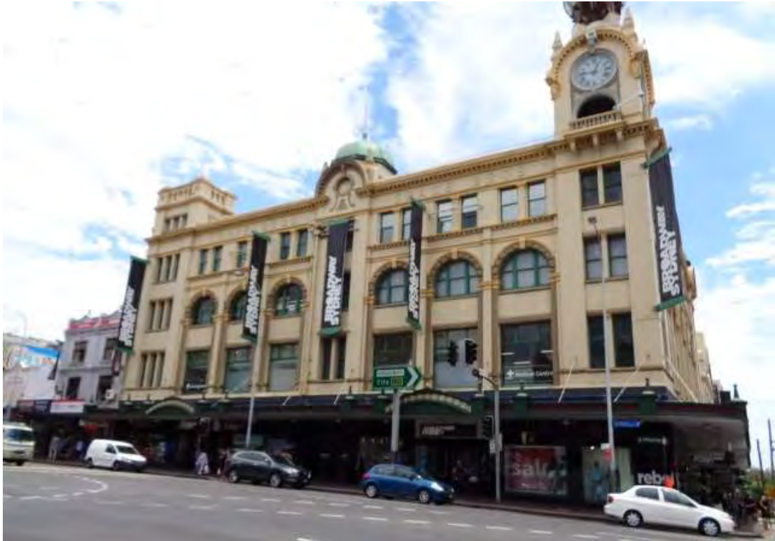
Figure 10: State heritage listed Former Grace Brother Building (Broadway Shopping Centre) to the east of the site on the corner of Broadway and Bay Street
