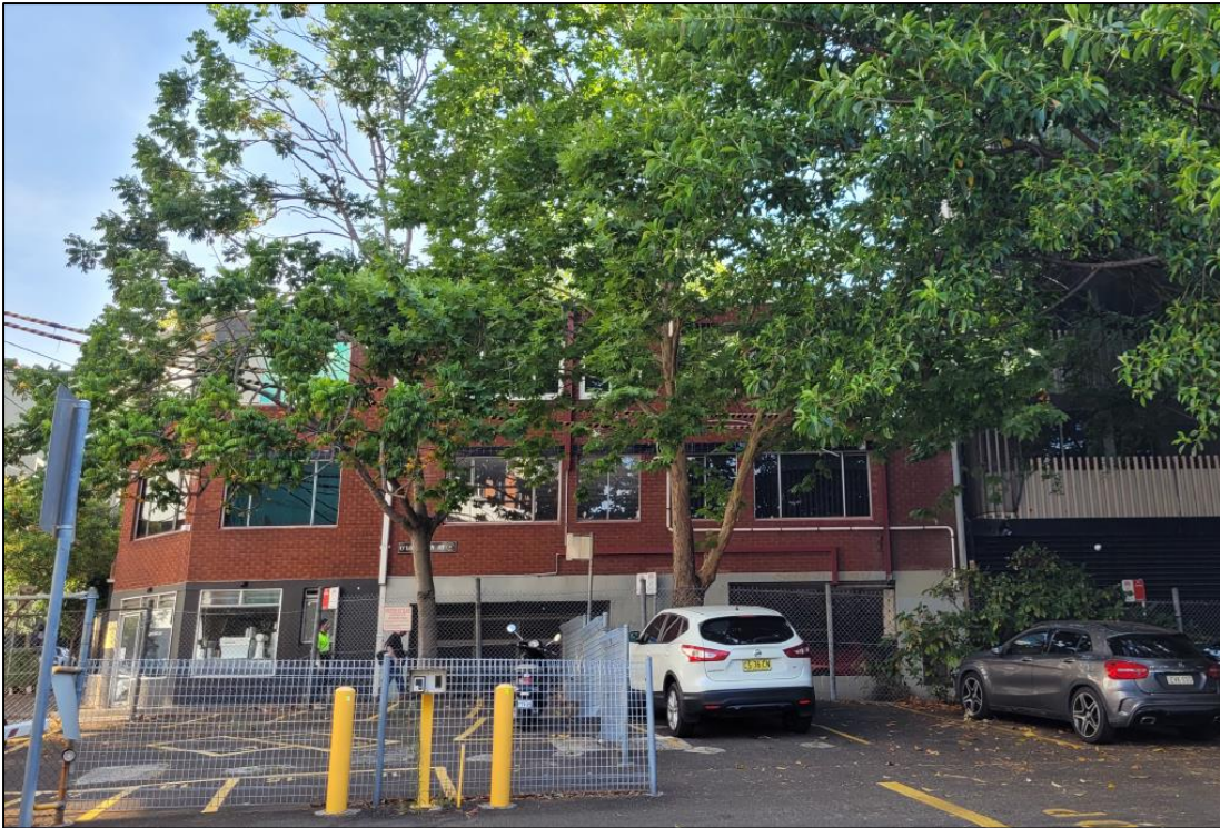
Figure 6: Site viewed from open carpark on the opposite side of O'Loughlin Street
