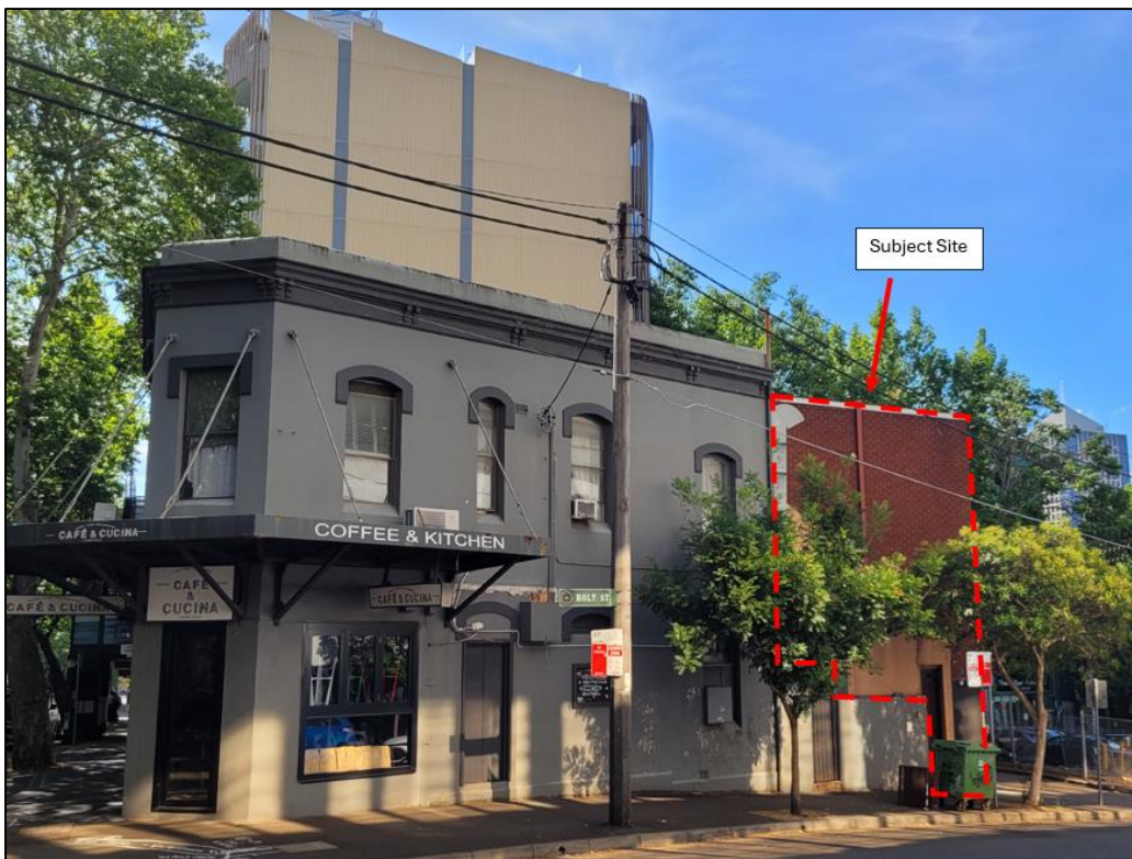
Figure 5: Site viewed from Holt Street looking west
