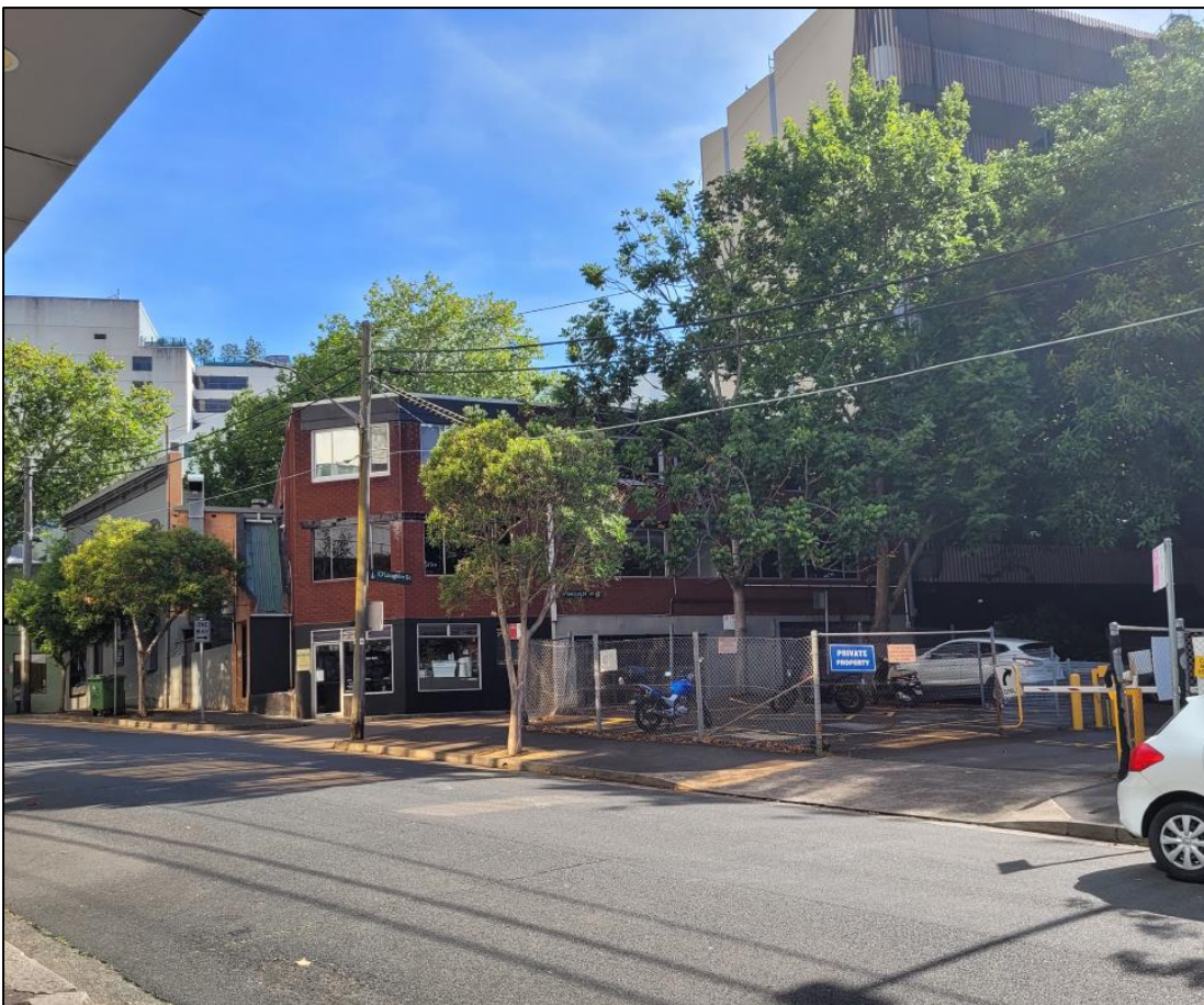
Figure 7: Site viewed from Holt Street looking south-west
