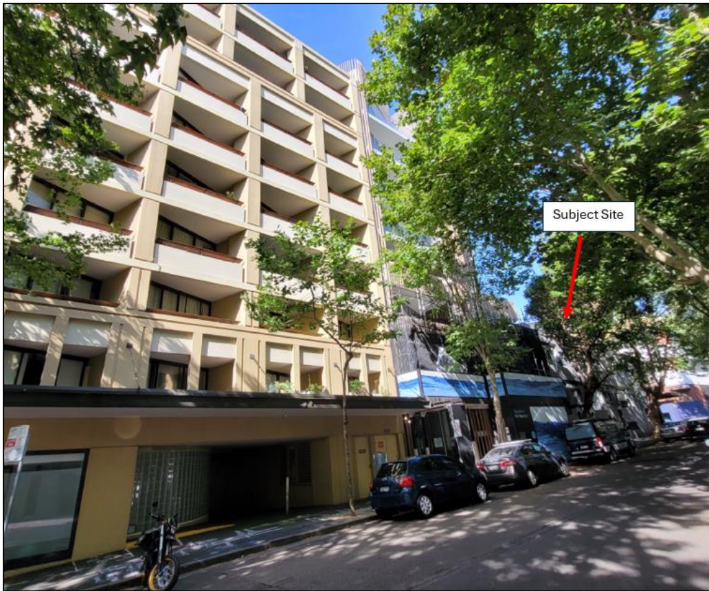
Figure 4: Site viewed from Cooper Street looking north-east
