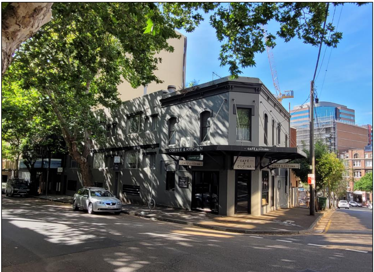
Figure 3: Site viewed from the corner of Cooper Street and Holt Street
