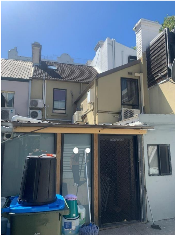
Figure 5: Rear of No. 43 Albion Street
