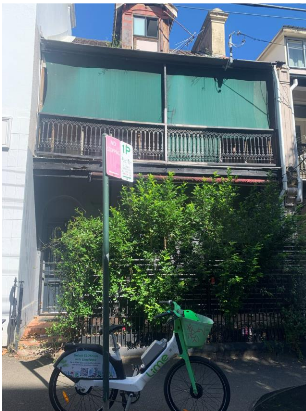
Figure 2: No.43 viewed from Albion Street. This property currently operates as a Brothel.
