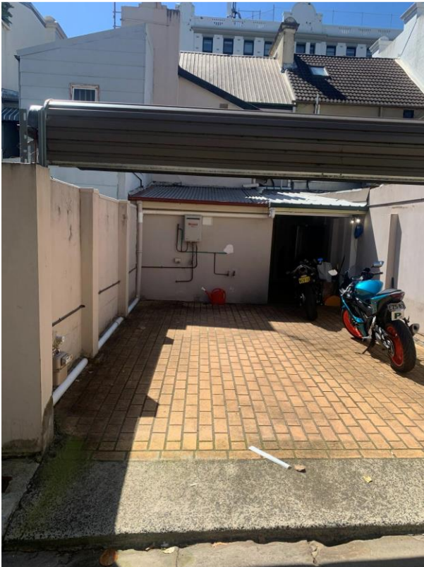
Figure 4: Rear of No.41 Albion Street, as viewed from Albion Way
