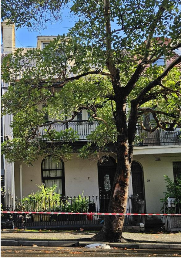
Figure 3: No.41 viewed from Albion Street
