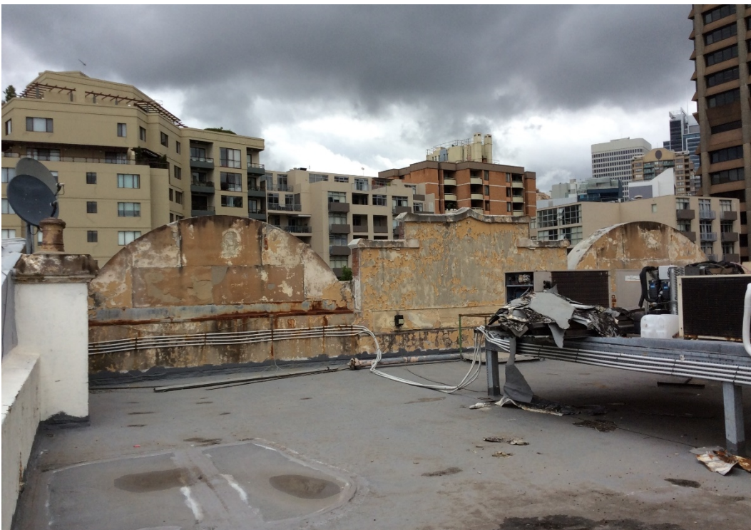
Figure 12: Existing rooftop and mechanical plant looking south
