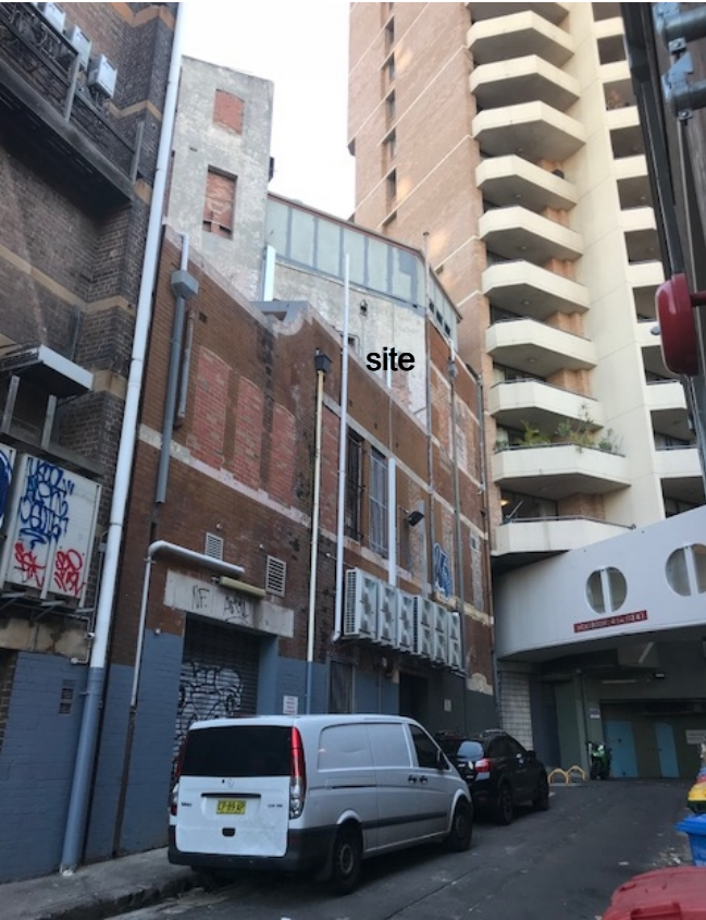
Figure 9: Rear of site viewed from Winns Lane
