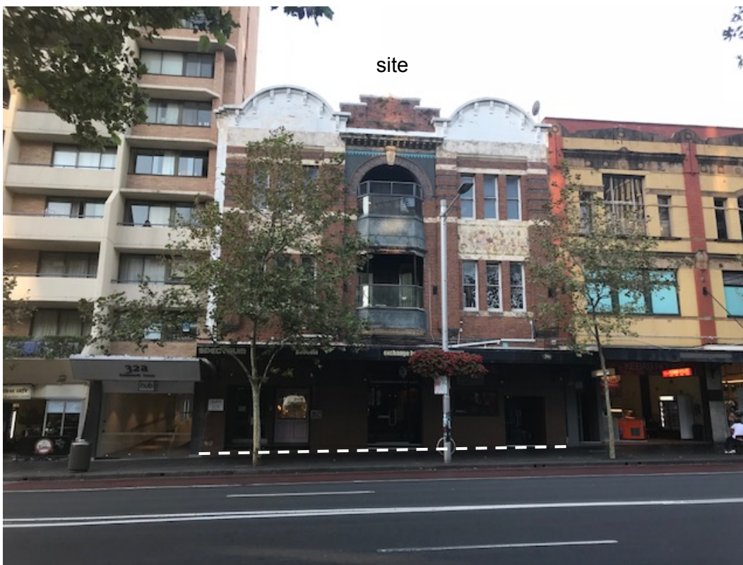
Figure 2: Site viewed from Oxford Street, looking north
