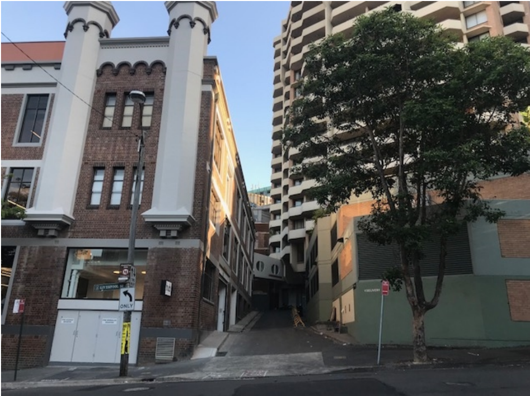
Figure 11: Site viewed from Liverpool Street looking south
