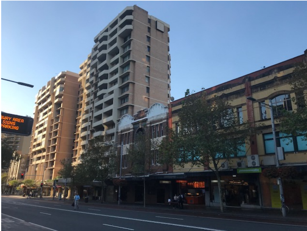
Figure 5: Looking north west along Oxford Street
