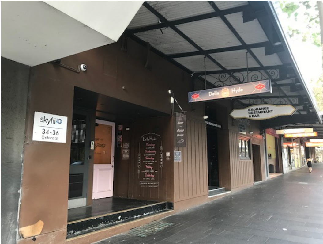
Figure 3: Existing ground floor facade
