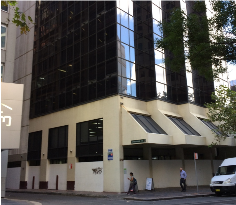
Figure 5: Site viewed from Pitt Street at corner of Underwood Street.
