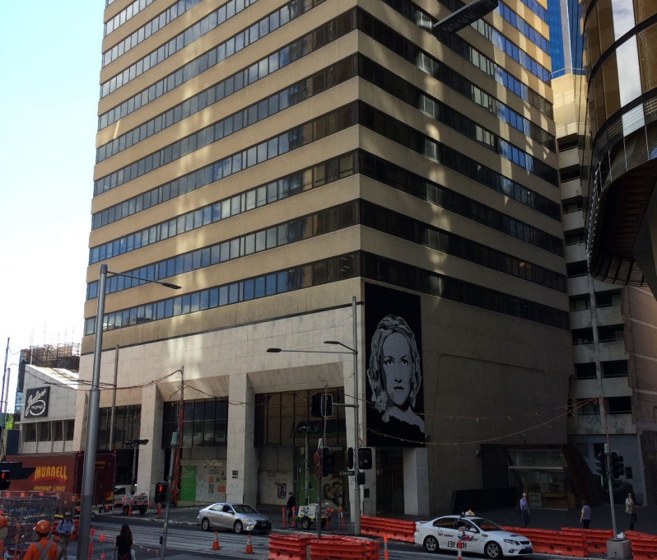
Figure 3: Site viewed from George Street looking east.
