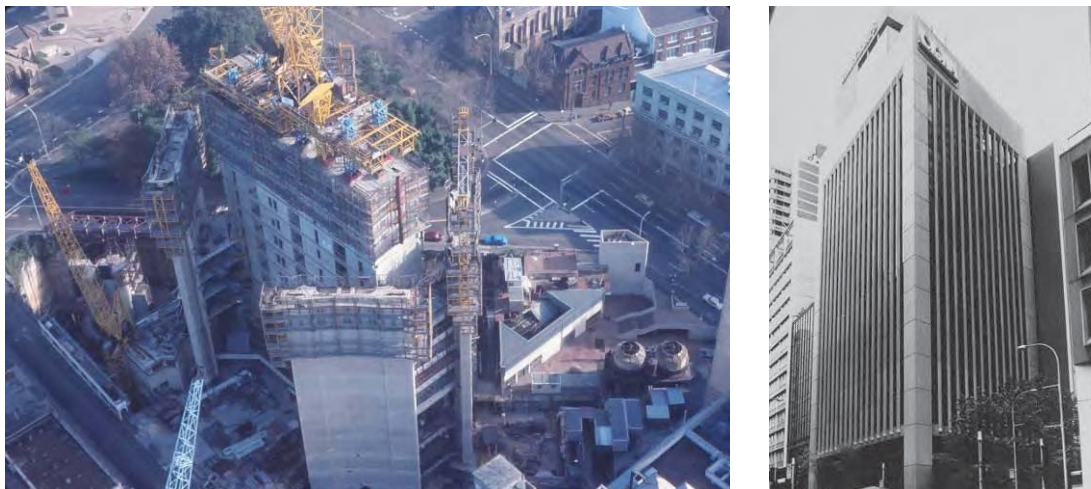
Figure 30 Second stage of the Qantas International Centre under construction, showing the relationship between the central core and the canted columns (left); former South British Insurance building in Hunter Street (right).
