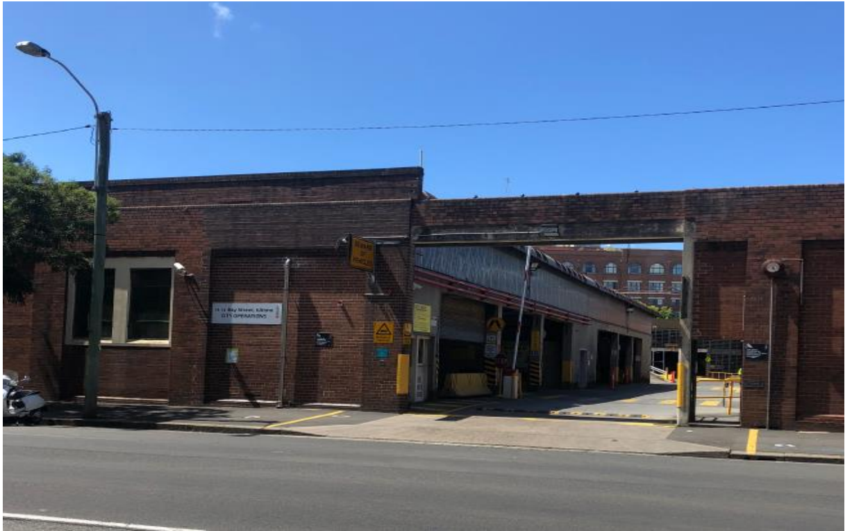
Figure 2: Site viewed from Bay Street with the garages building located within the site, and visible to the left of the opening
