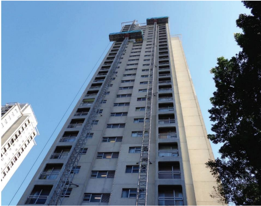
Fig 8. Existing towers undergoing façade resealing.
