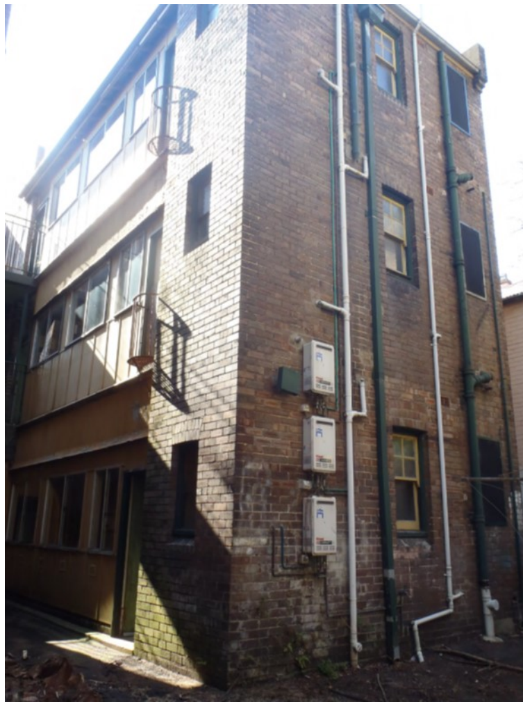
rear of no. 30
