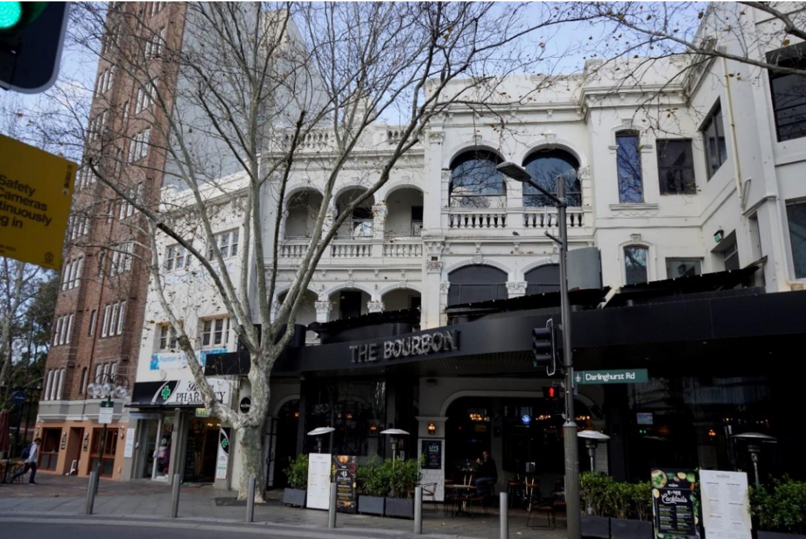
Figure 4: The facade of The Bourbon at 22-24 Darlinghurst Road, Potts Point
