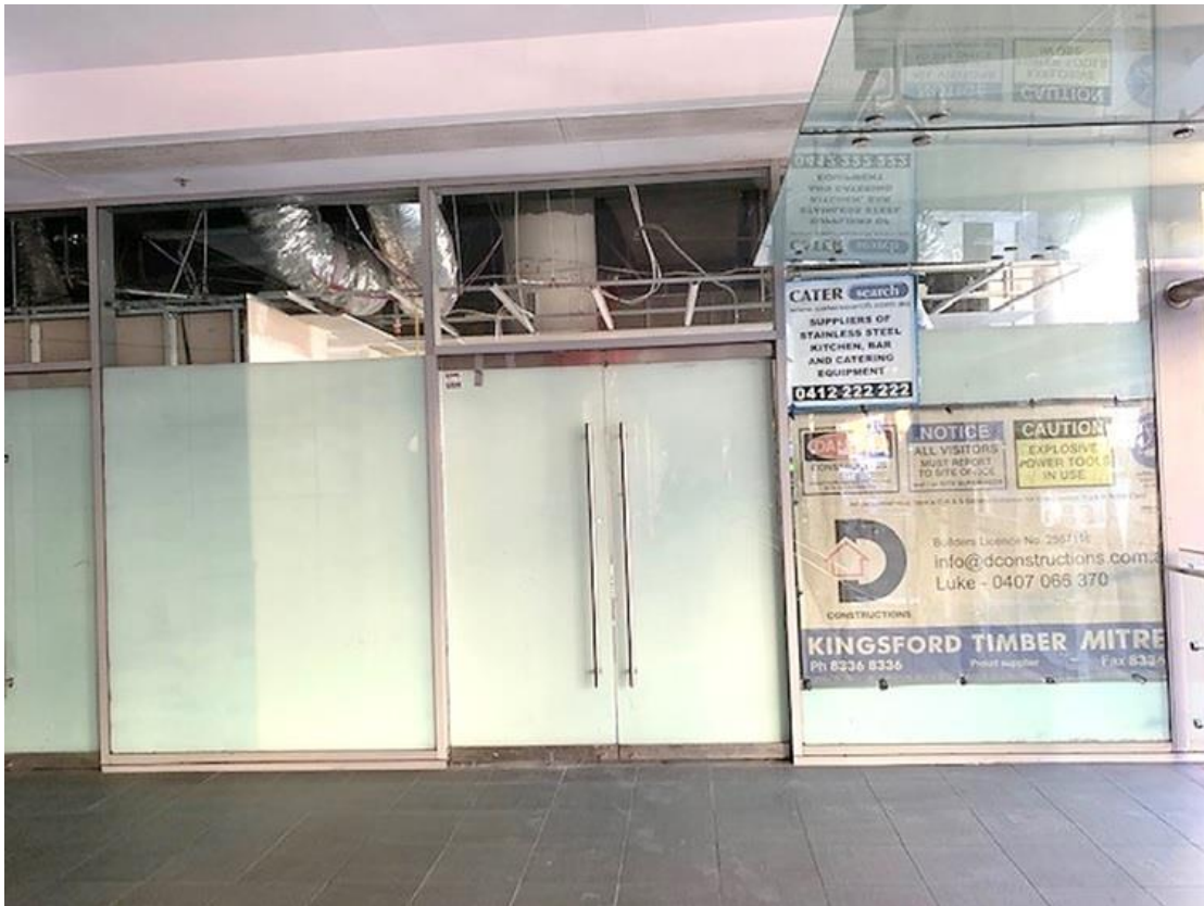
Figure 4: Existing shopfront (proposed to be altered).
