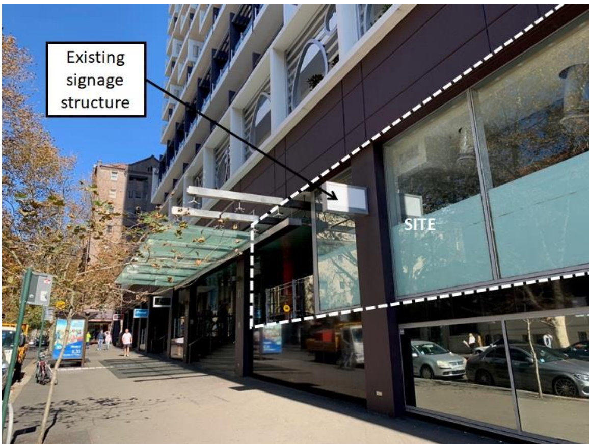
Figure 3: Existing signage structure (signage content proposed to be replaced).
