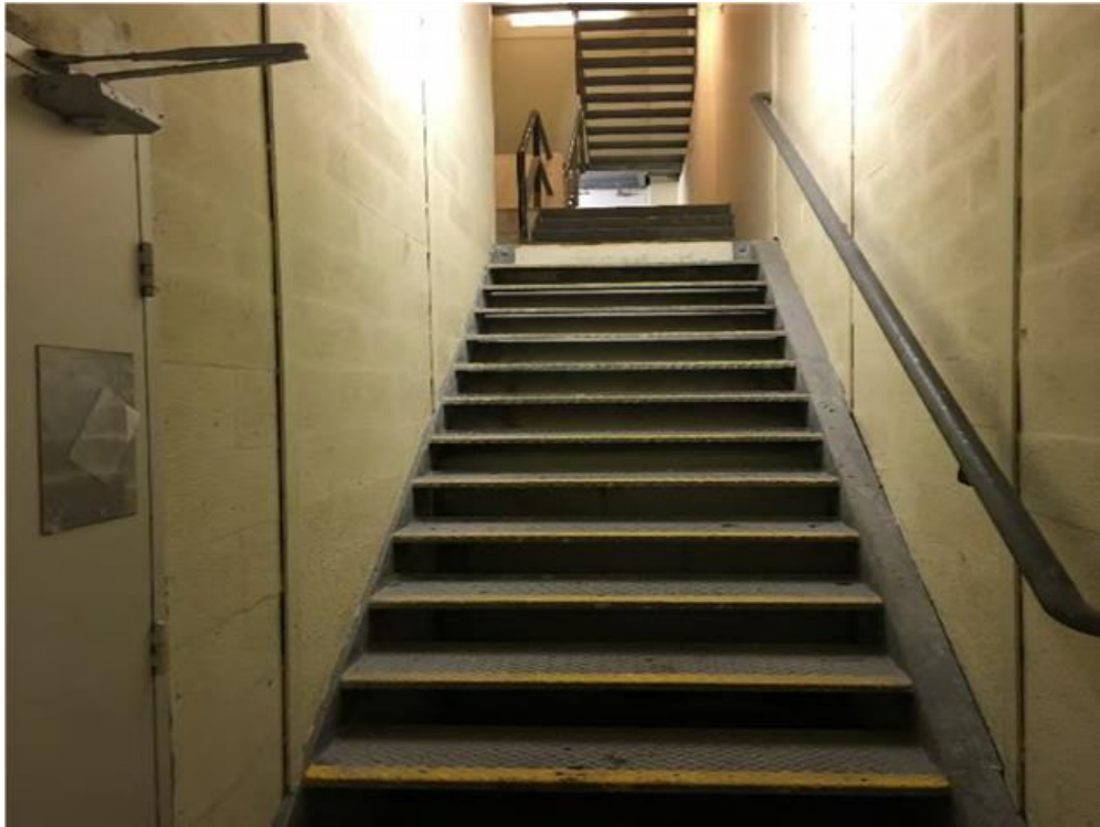
Figure 36: The eastern light well at 198-200 Pitt Street partially infilled for a fire stair.
