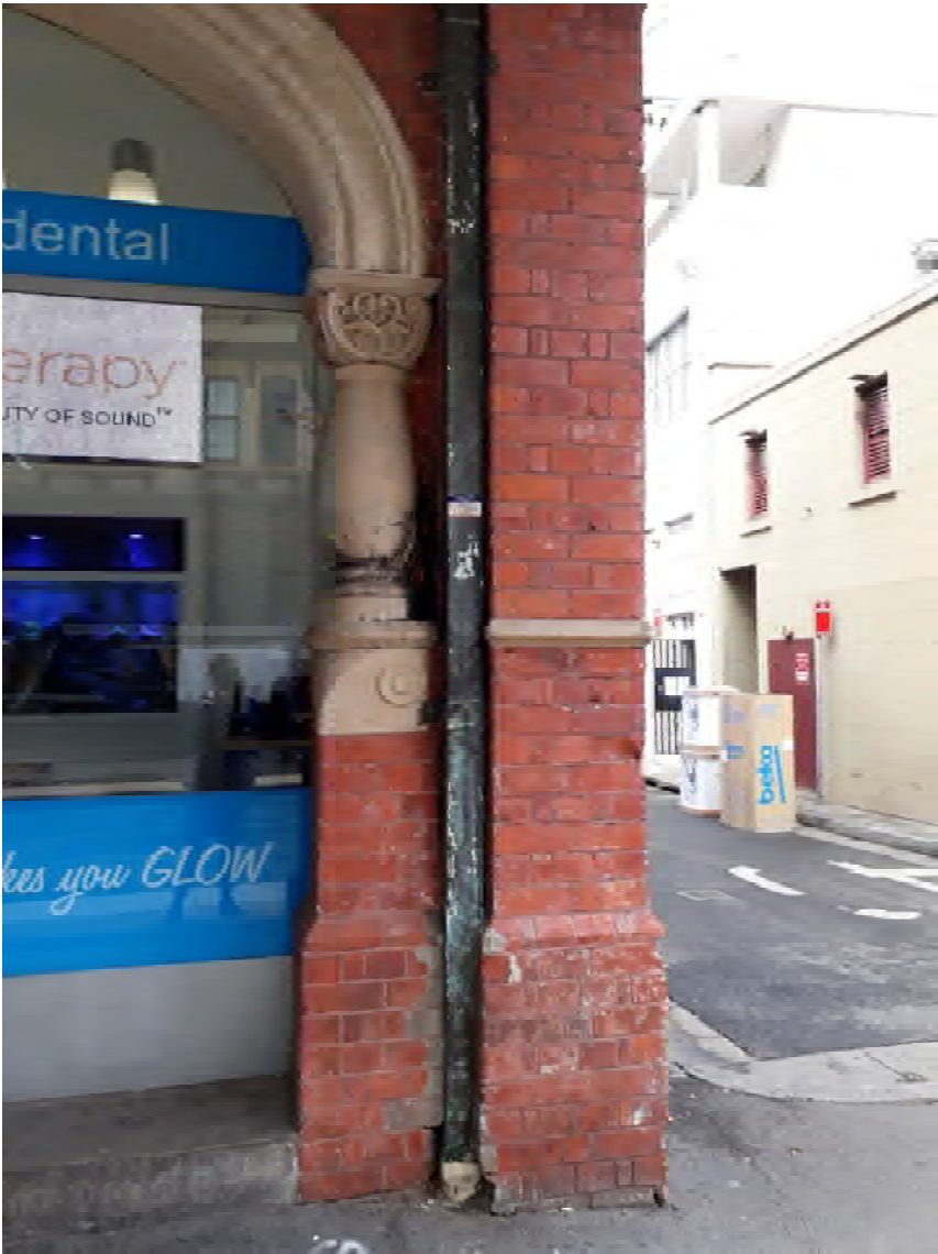
Figure 14 – Defect 16 – impact damage to maosnry
