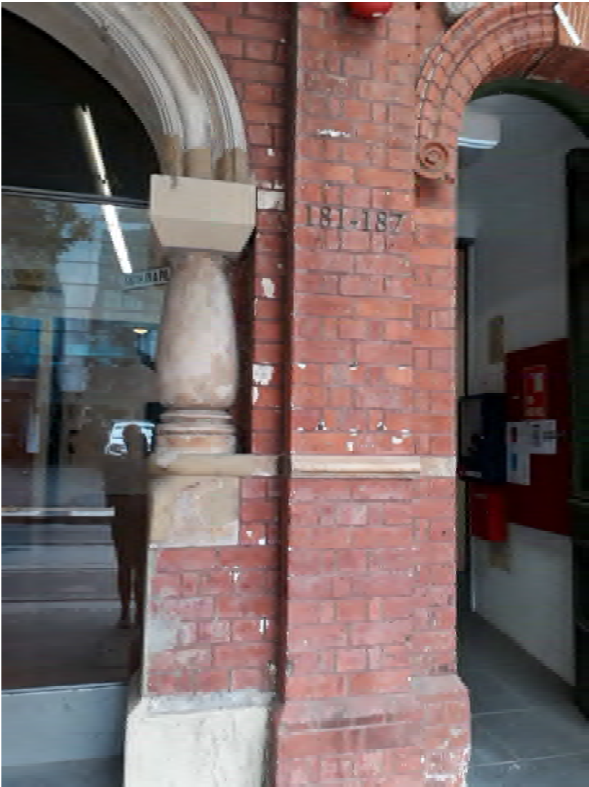
Figure 13 – Defect 15 – previous repairs to masonry
