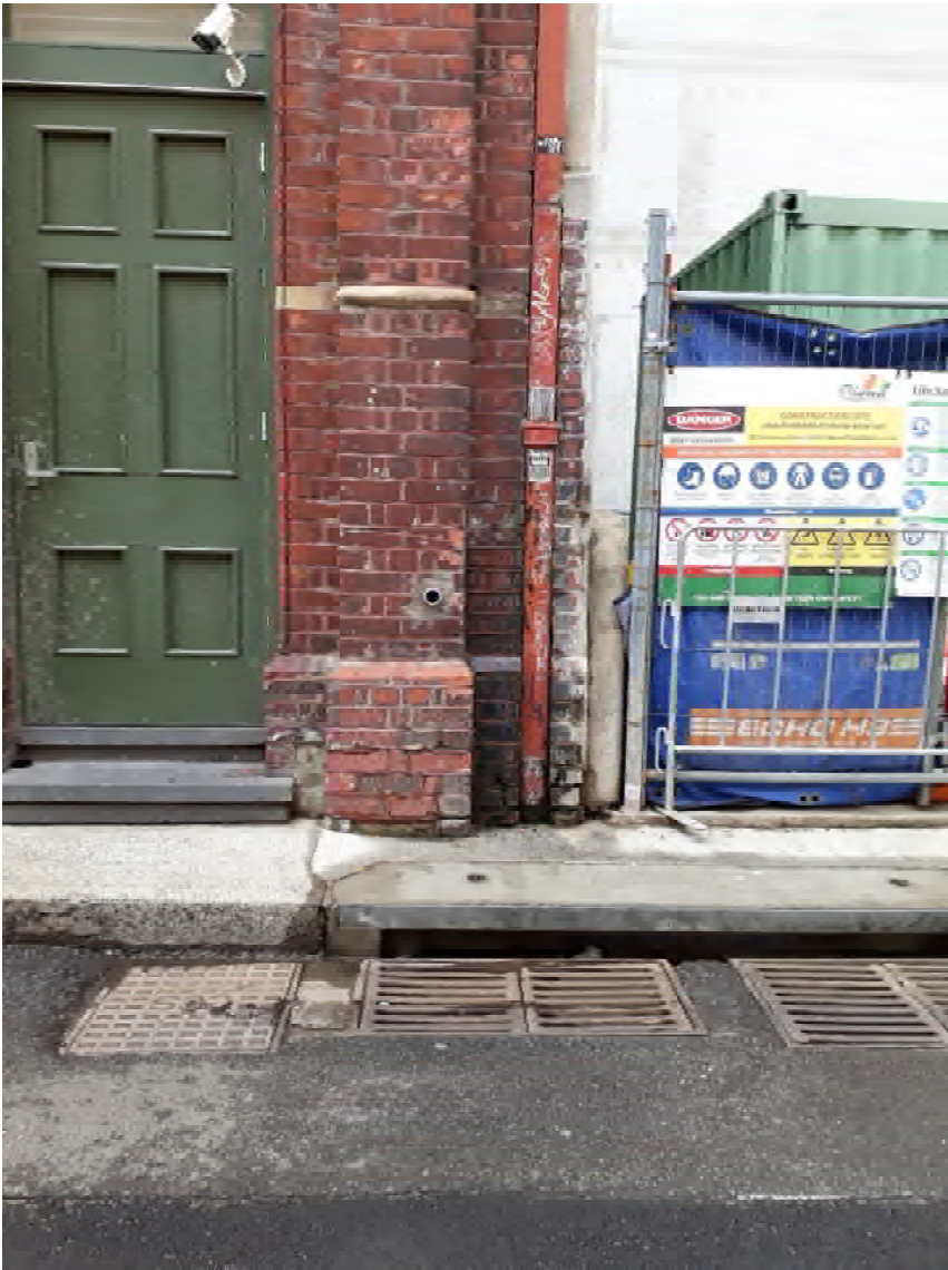
Figure 16 – Defect 18 – damp masonry
