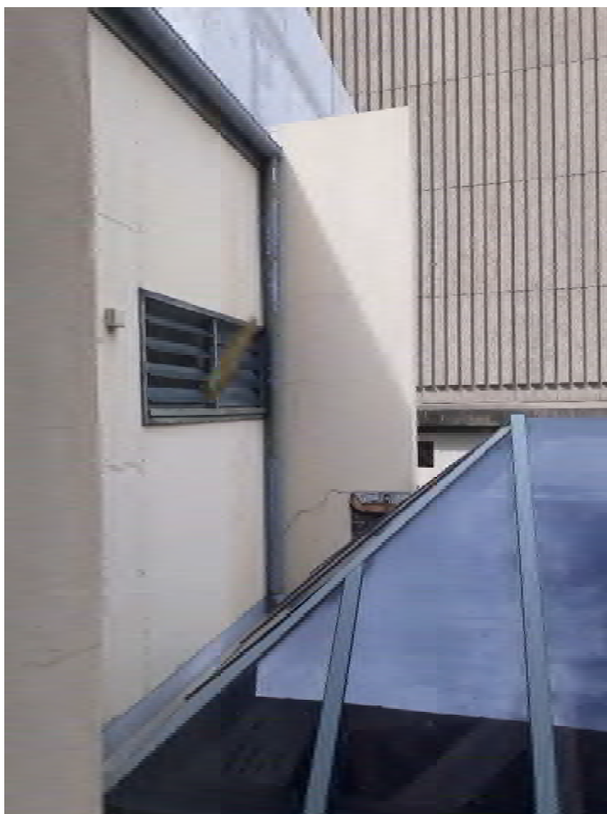
Figure 3 – Defect 4 – cracks in masonry
