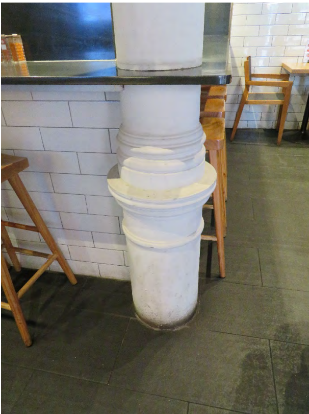
Figure 78 – Cast iron column in dining area of Tenancy 4
