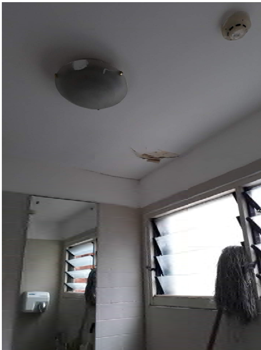
Figure 1 – Defect 1 - Water damage.
