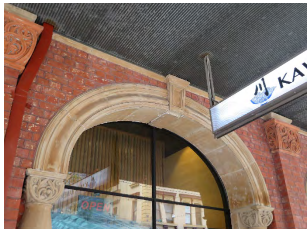
Figure 81 – Discoloured sandstone arches
