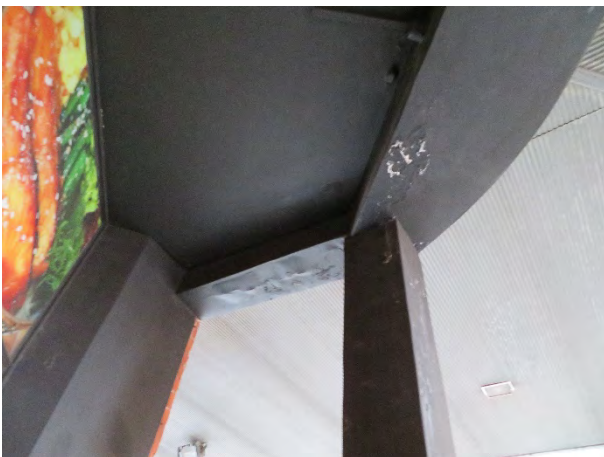
Figure 80 – Damp issues on ground floor corner entrance.
