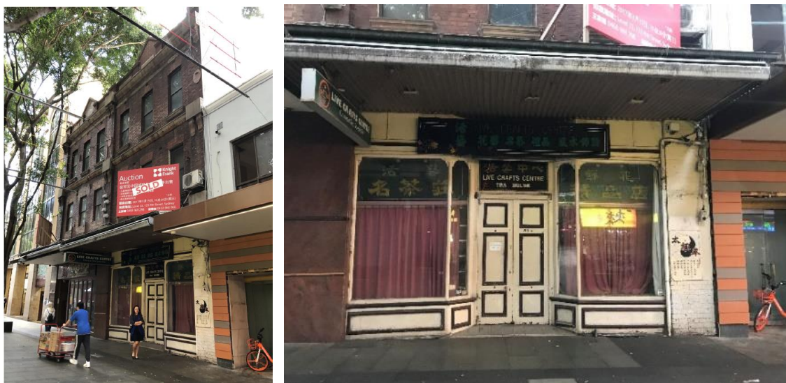
Figure 2: Subject building at 82-84 Dixon Street, with 84 Dixon Street shopfront on right.
