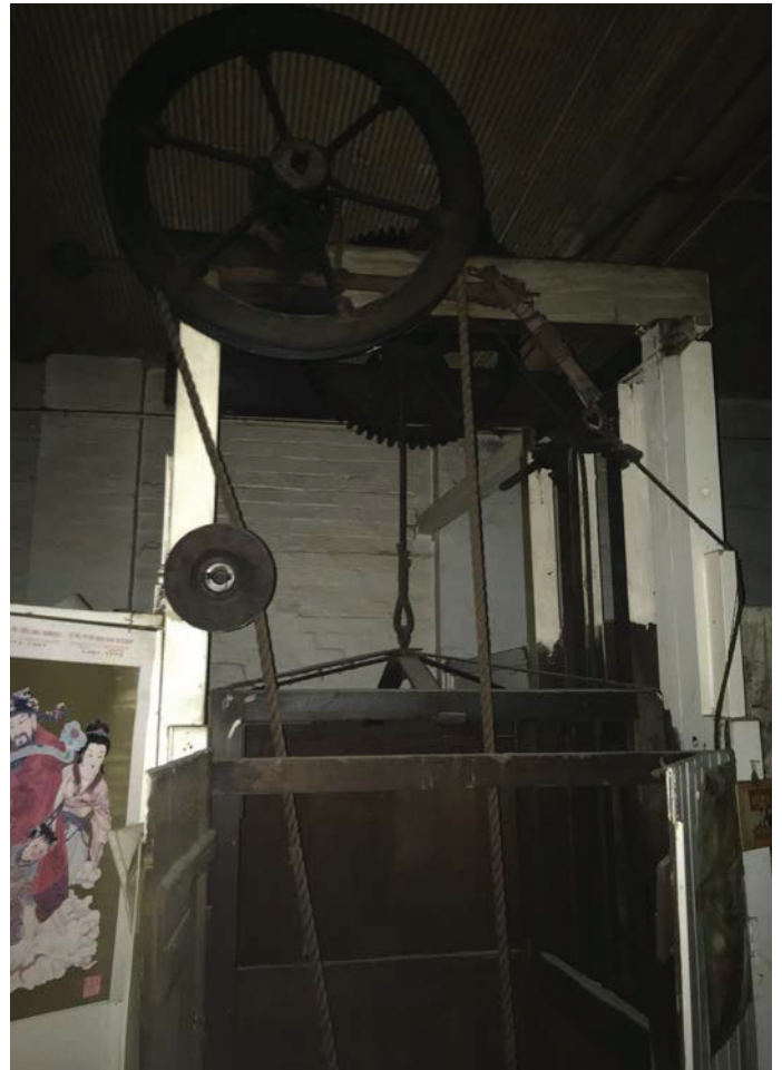
Figure 4: Goods lift mechanism.
