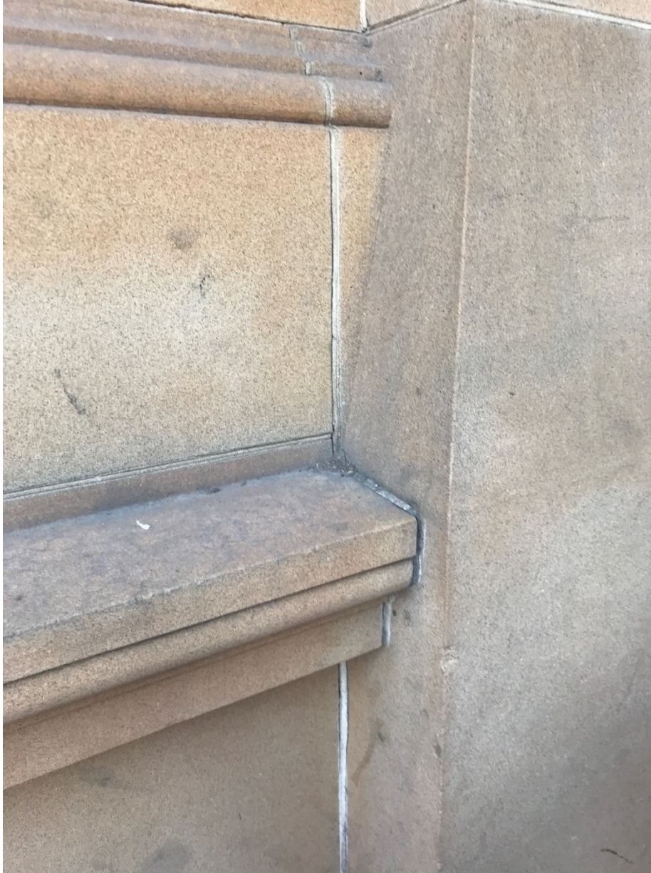
Figure 1 – Loose and missing exterior pointing.
