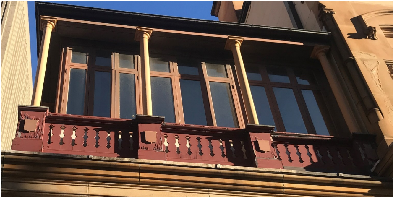
Figure 3 – Paint flaking on timber of enclosed veranda.
