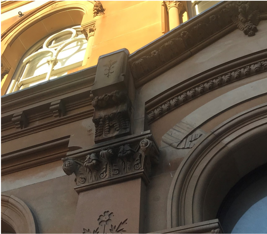
Figure 6 – Polluted water running over brackets on either side of front door.
