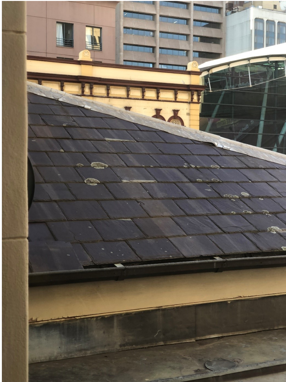
Figure 8 – Slate has slipped on veranda roof, lead hip flashing is lifting.
