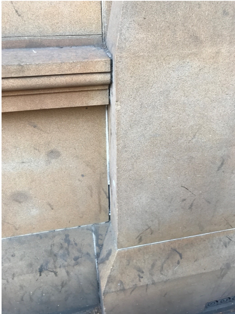
Figure 2 – Superficial dirt on lower courses of stonework
