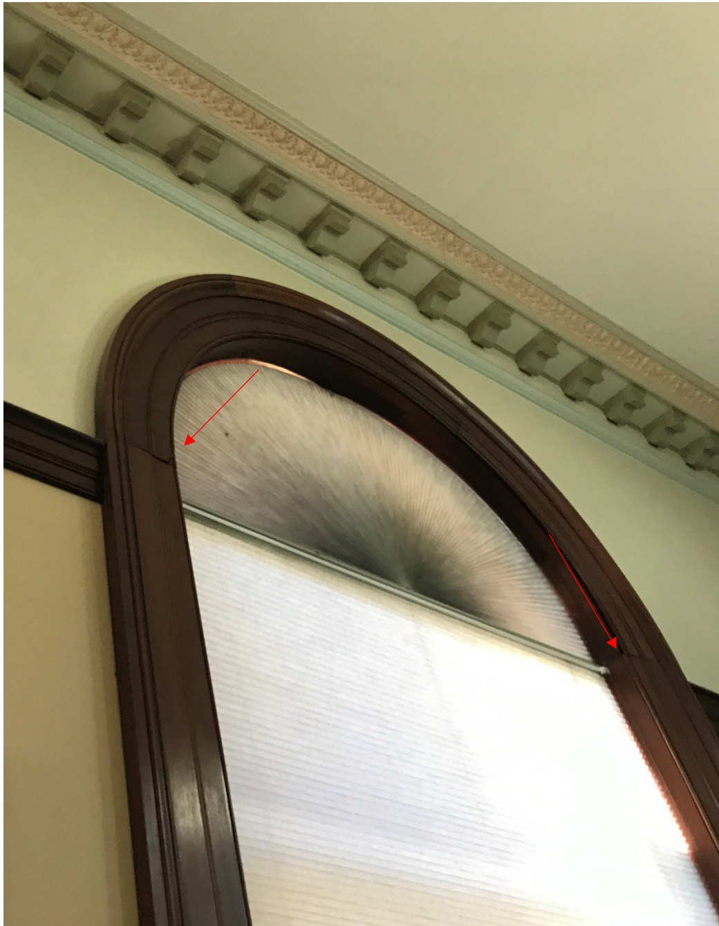
Figure 9 – Architraves misaligned where vertical meets rounded section, likely due to movement.
