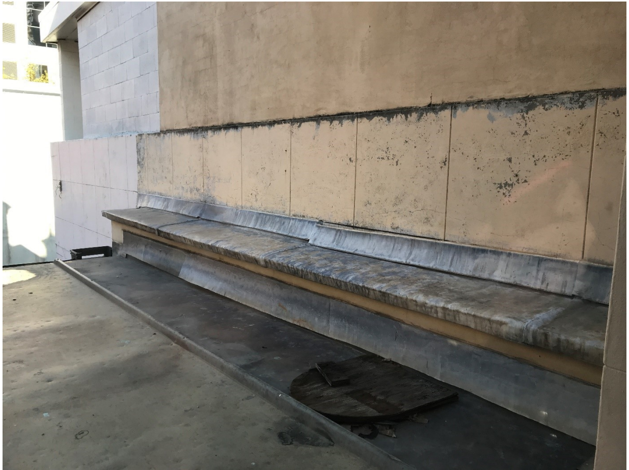
Figure7 – Apron flashing on southern boundary wall has slipped.
