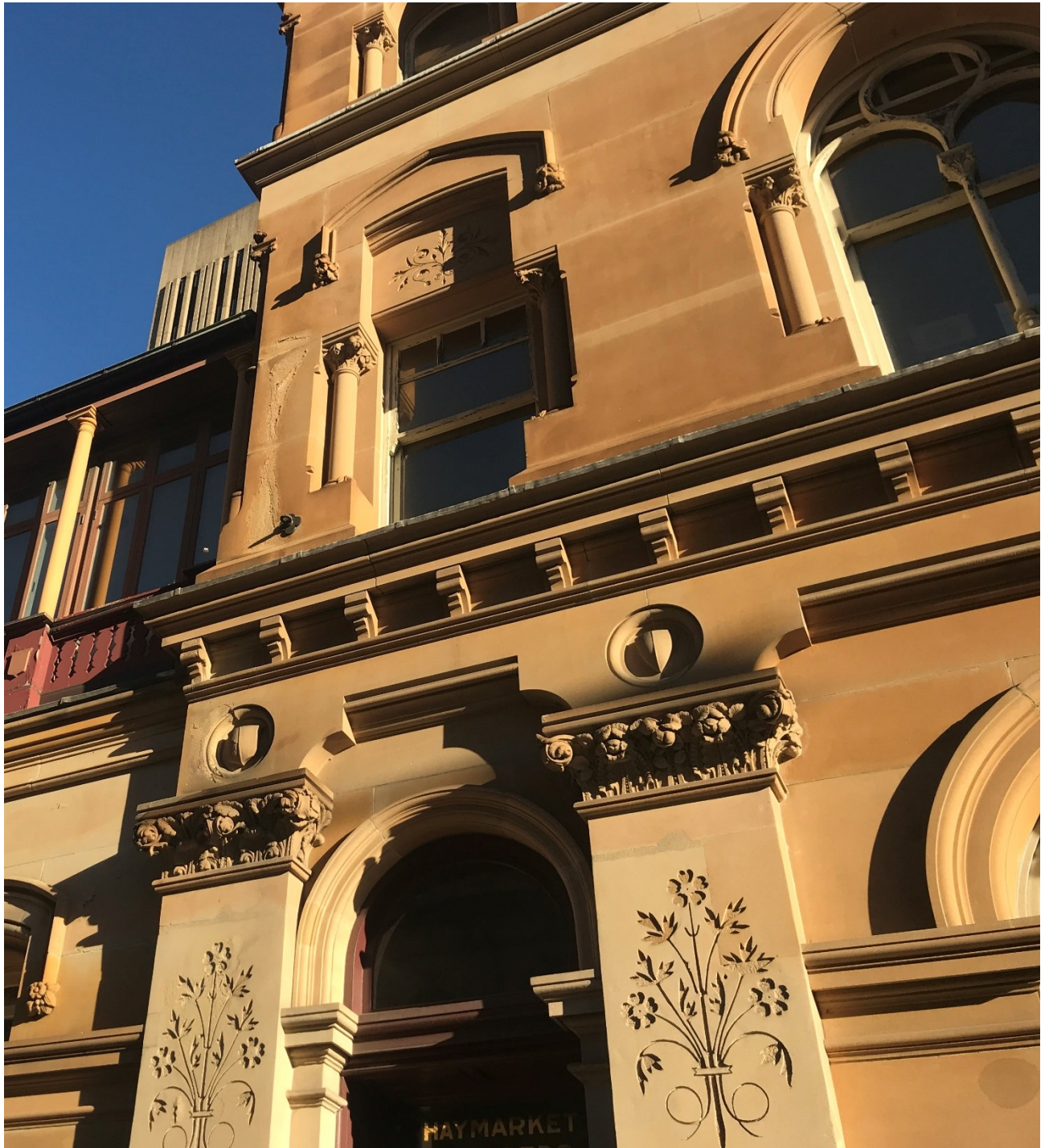
Figure 4 – Lateral damp affecting stonework at eastern end of north façade, possibly failing.
