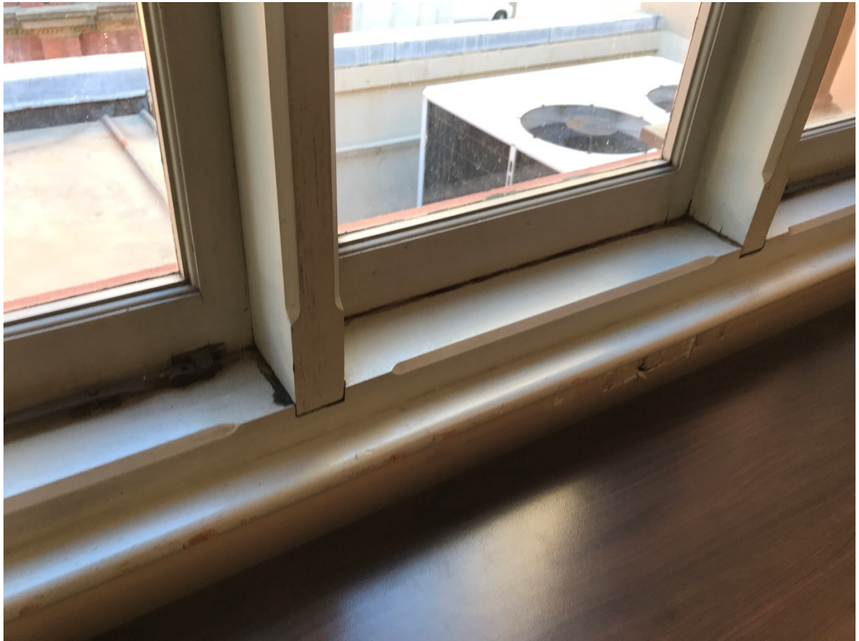
Figure 10 – Signs of leaking window sills in glazed veranda.
