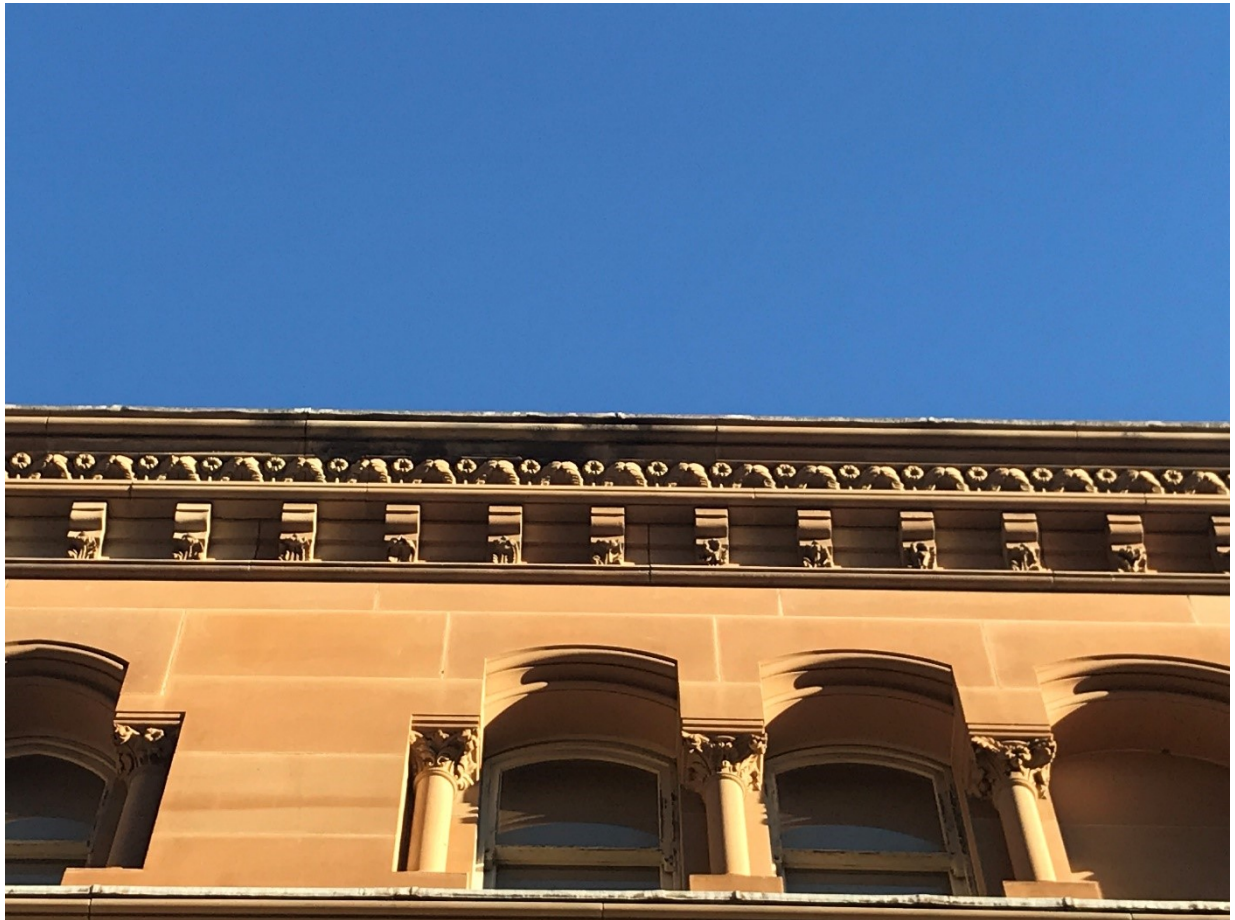
Figure 5 - Evidence of water and active decay in cornice on north façade. Lead lifting off coping.
