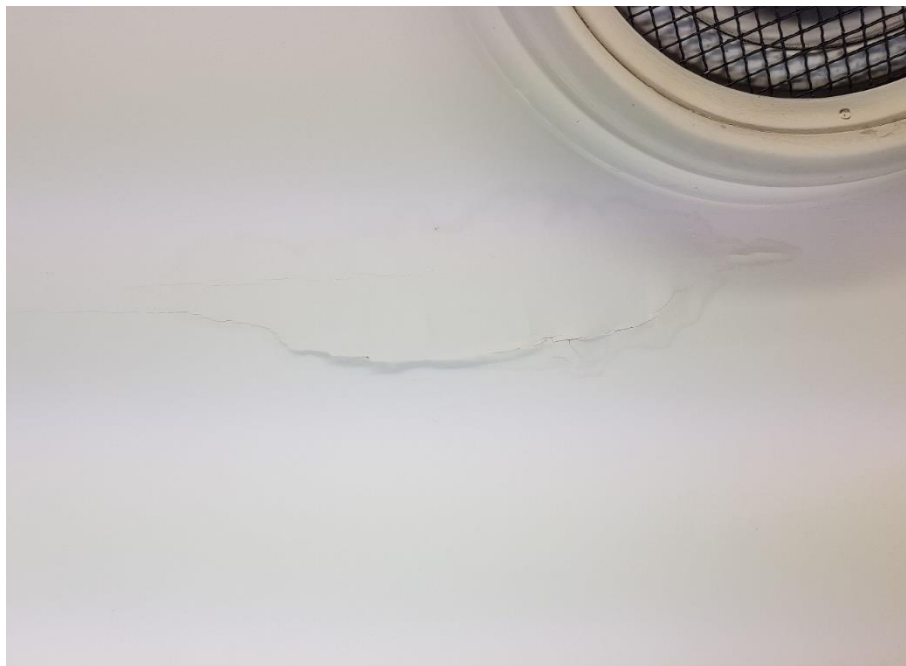
Figure 1: Leak Through Ceiling Near Air Conditioning Vent
