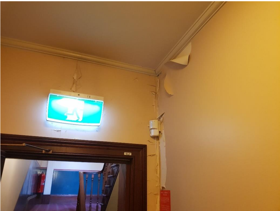
Figure 4: Leak in Roof at Stair Landing Level
