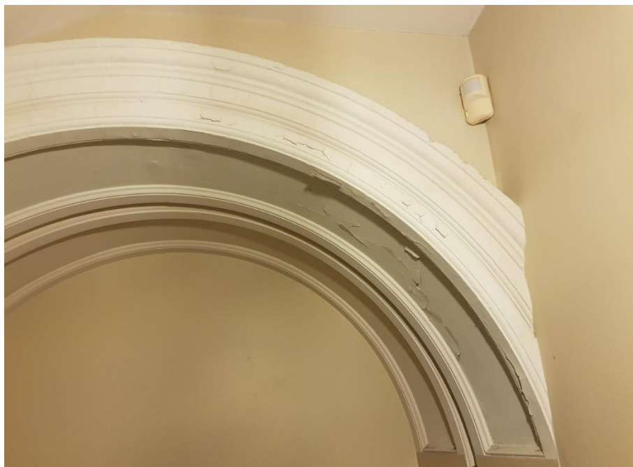
Figure 2: Cracked Paint Around Arch, Non-Structural
