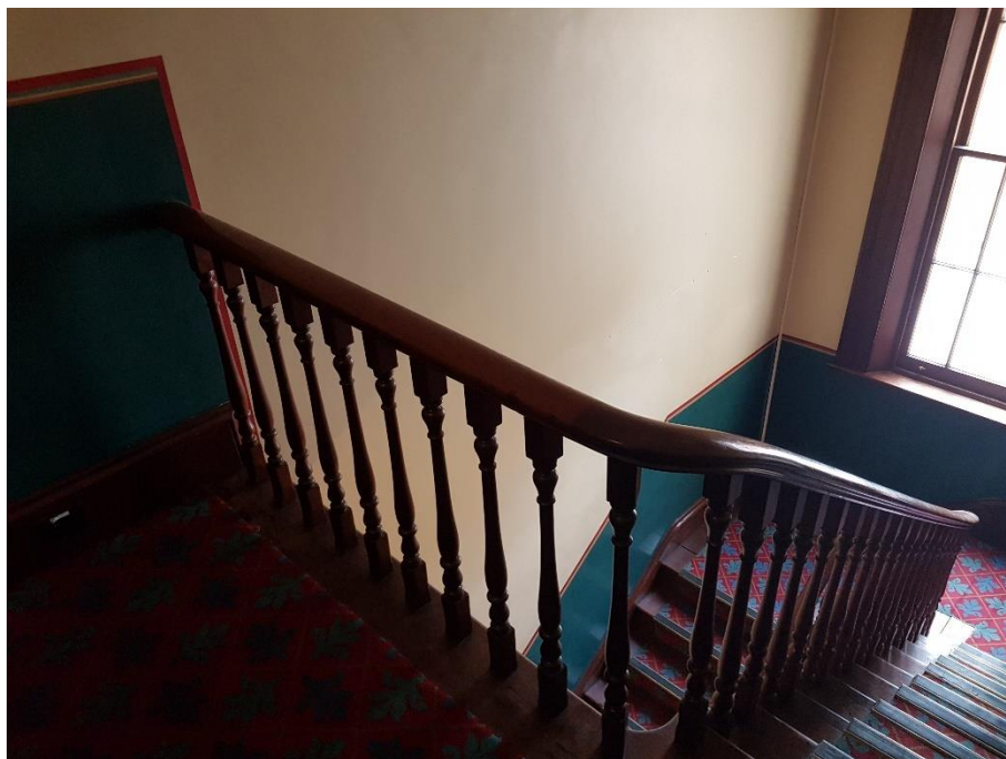
Figure 11: Low Balustrade to Landing 800mm High
