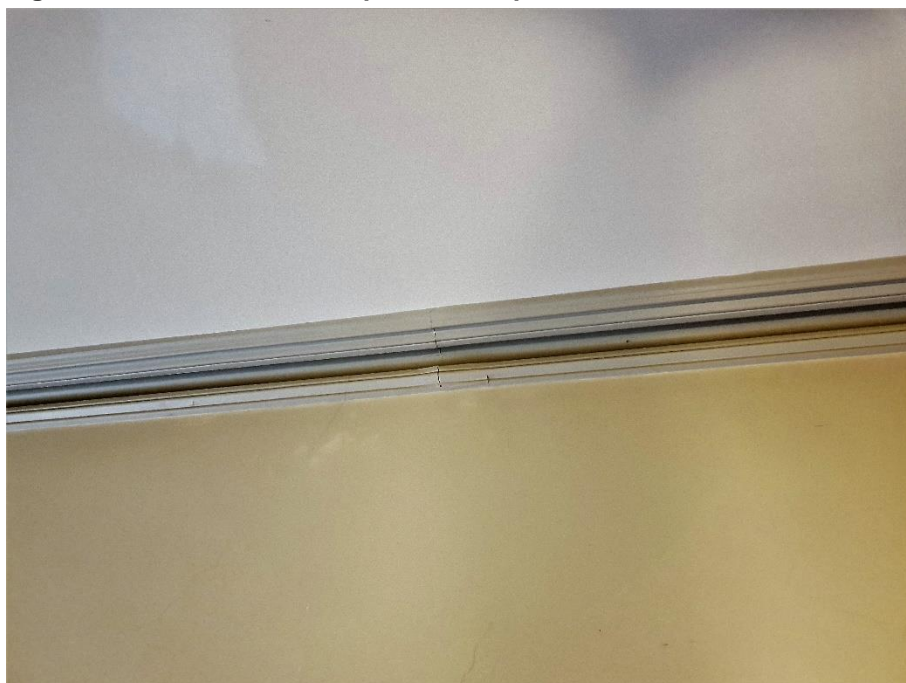
Figure 12: Cornice Crack Repaired Multiple Times
