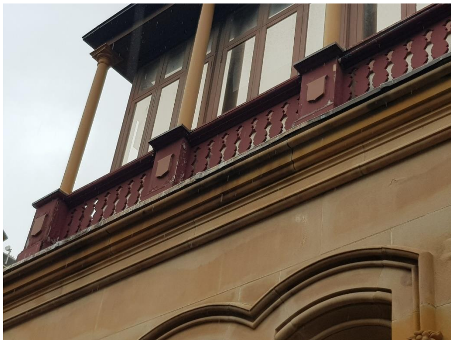
Figure 13: Timber Paint Peeling
