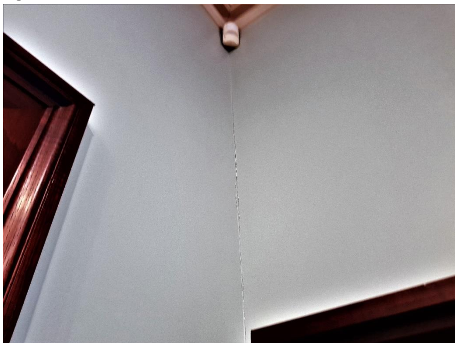
Figure 8: Crack in Corner
