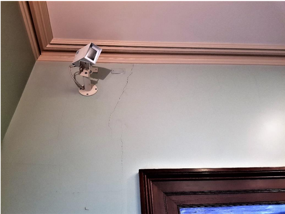
Figure 9: 2mm Cracking Over Door, Crazed Cracking
