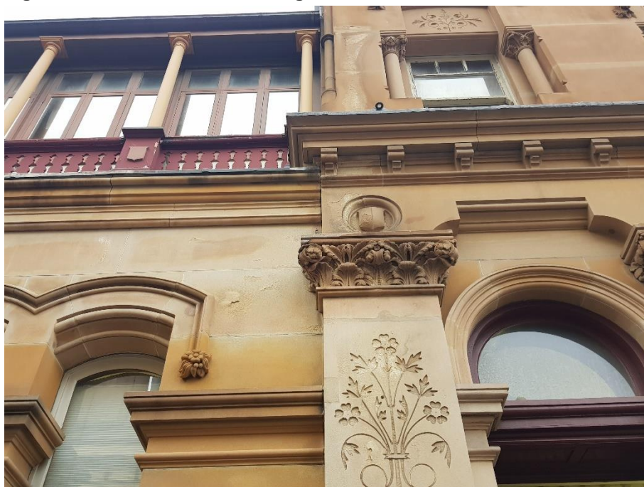
Figure 14: Sandstone Weathering
