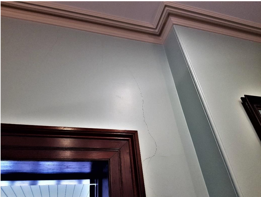
Figure 10: 2mm Cracking Over Door, Crazed Cracked
