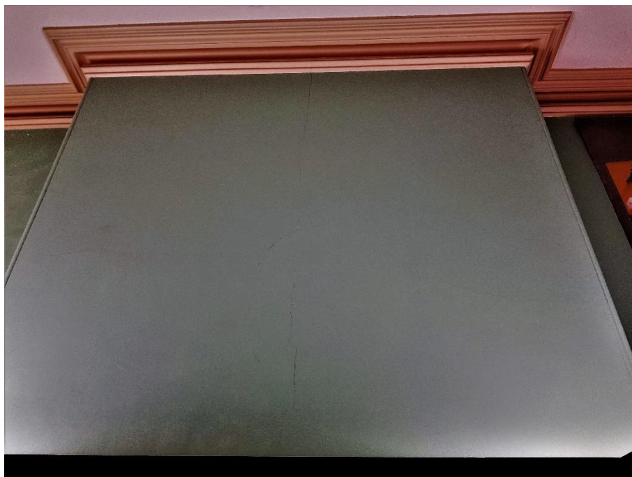
Figure 5: Minor Cracking on Chimney Breast ~1mm
