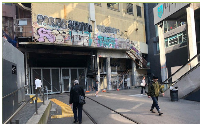
Figure 10 Existing End of Goods Line shows the potential tunnel to Central (Source HillPDA)
