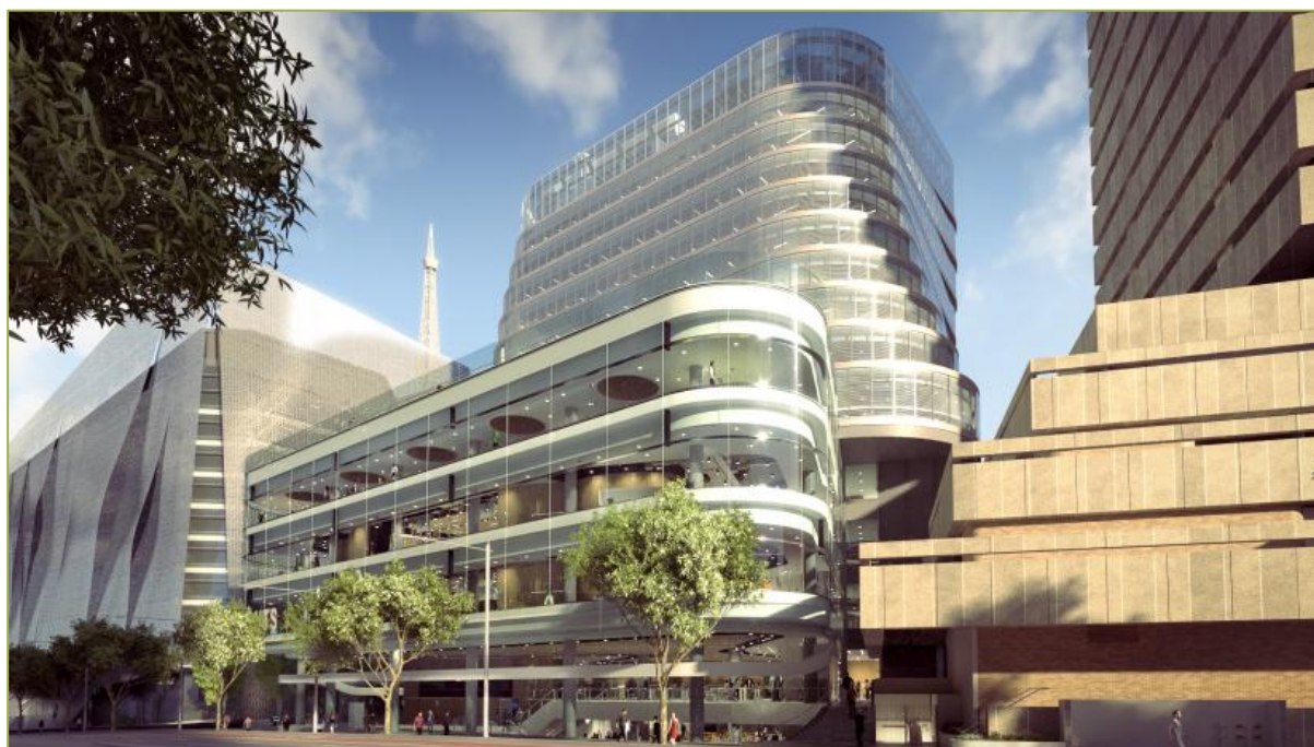
Figure 6: UTS Campus Building 2 Open Plan Collaborative Space & Library
