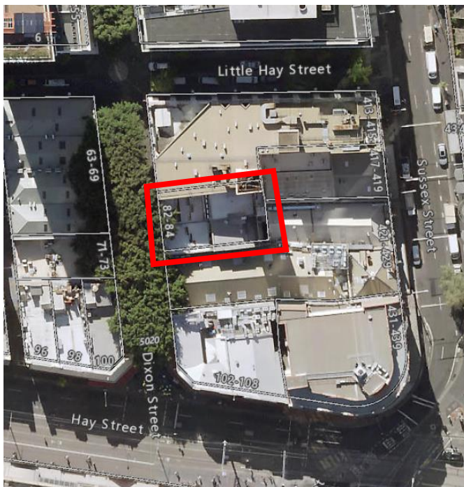
Figure 1: Site of 82-84 Dixon Street
