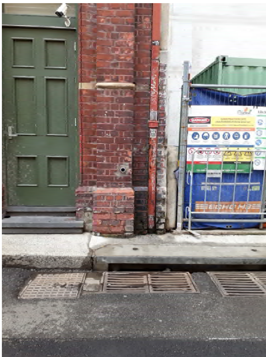
Figure 16 – Defect 18 – damp masonry
