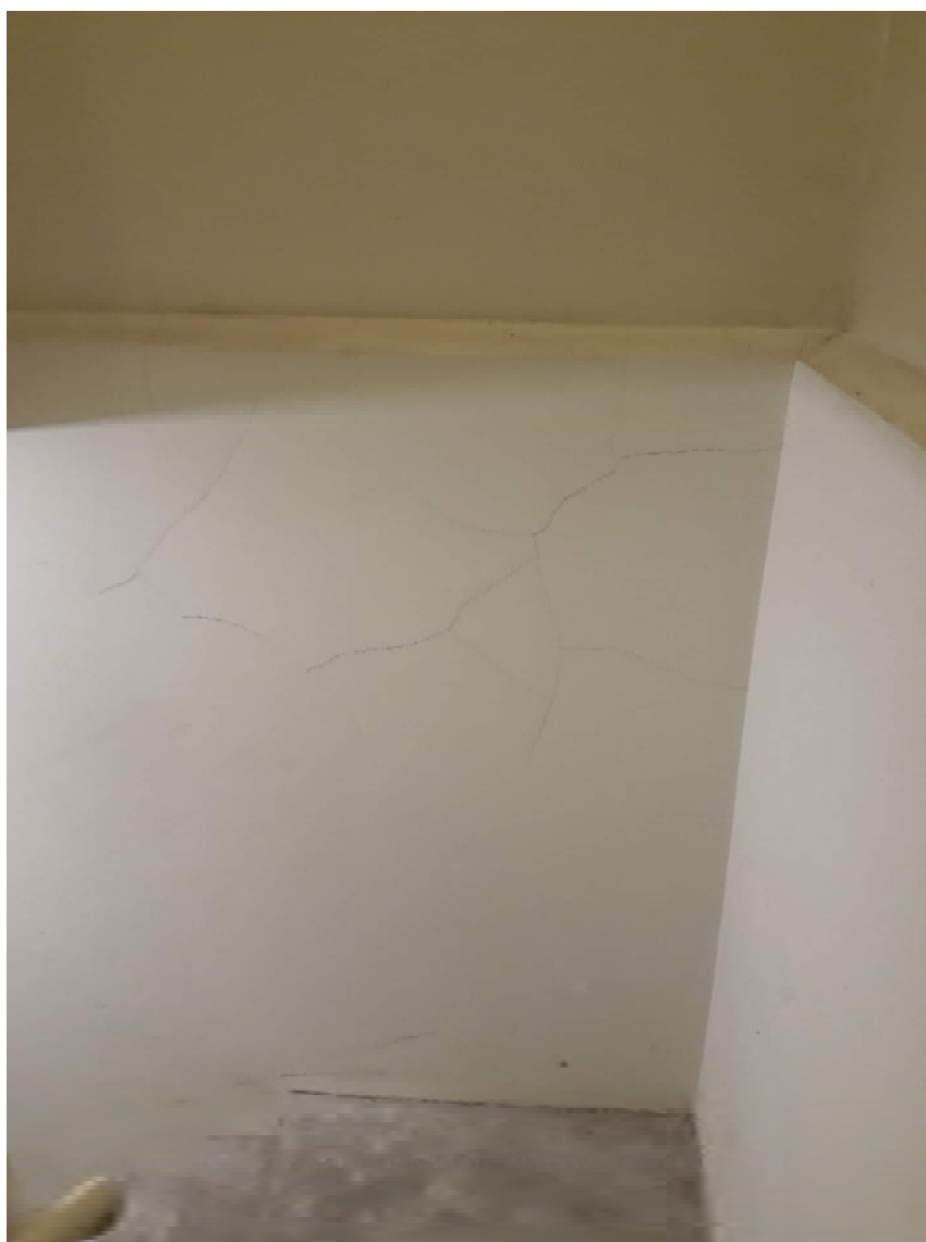
Figure 2 – Defect 3 – cracks in masonry
