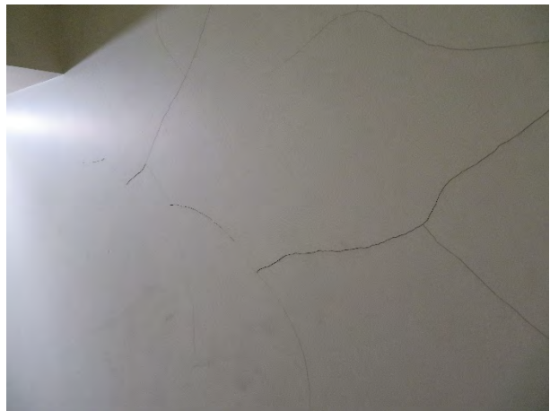
Figure 85 – Cracks in southern wall of fire stair
