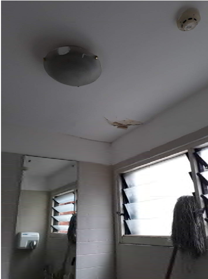
Figure 1 – Defect 1 - Water damage.
