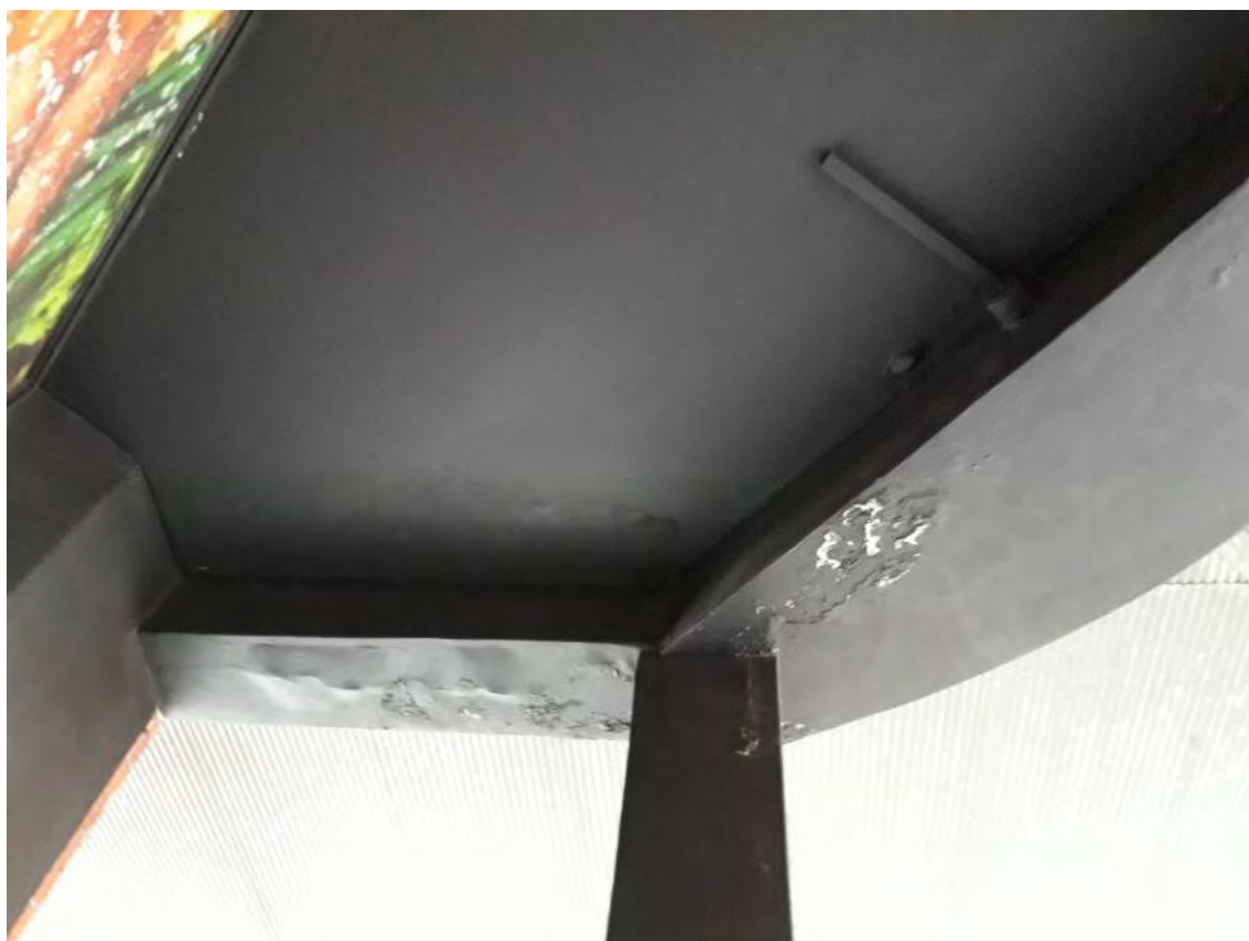
Figure 7 – Defect 8 - damp
