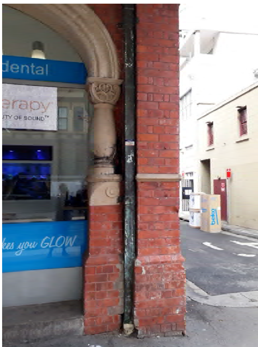
Figure 14 – Defect 16 – impact damage to maosnry
