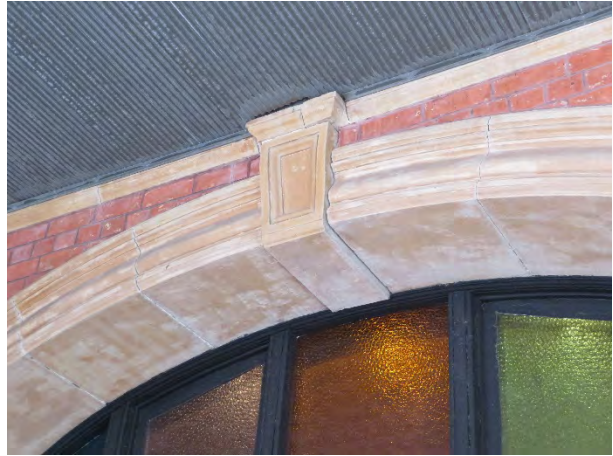
Figure 28 – Keystone detail of sandstone arch on Parker Street
