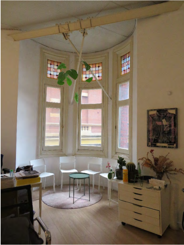
Figure 68 – Steel beam and tie rods for awning support in turret on first floor of Tenancy 3
