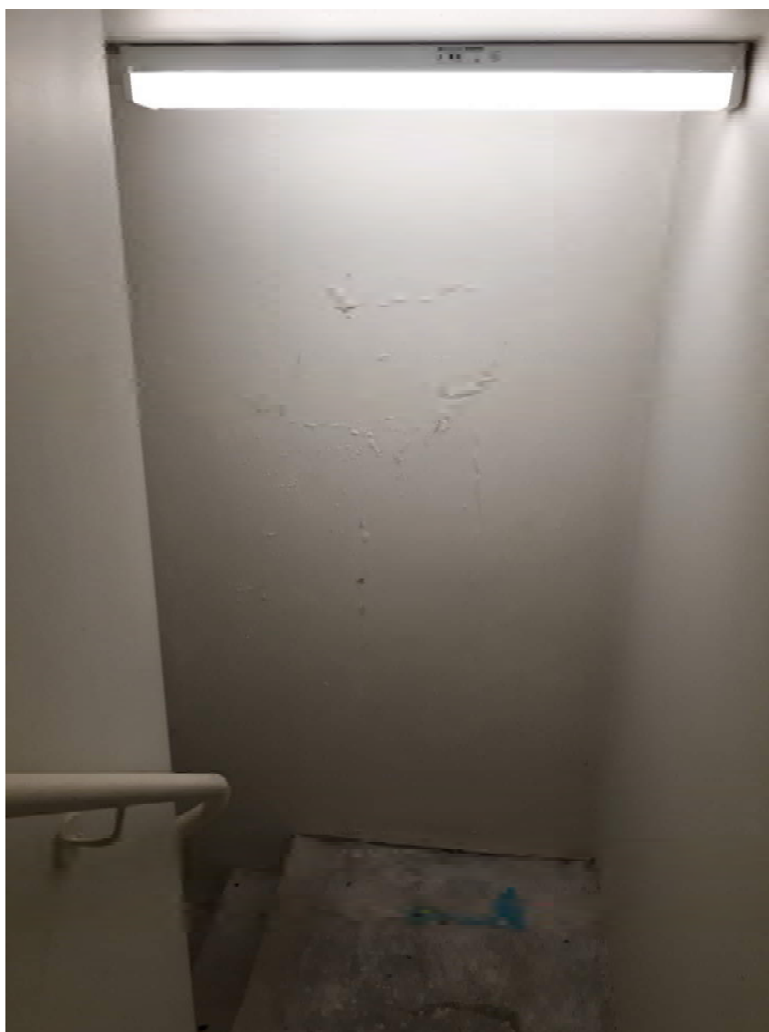
Figure 4 – Defect 5 - damp
