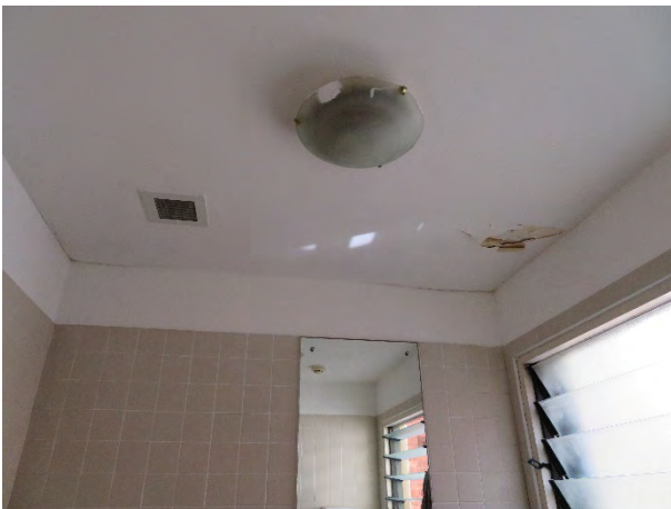
Figure 84 – Water damage in disabled toilet on first floor
