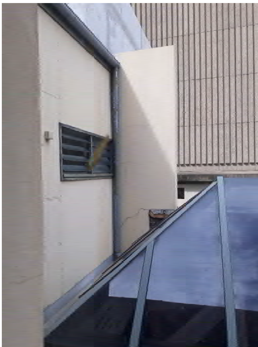
Figure 3 – Defect 4 – cracks in masonry
