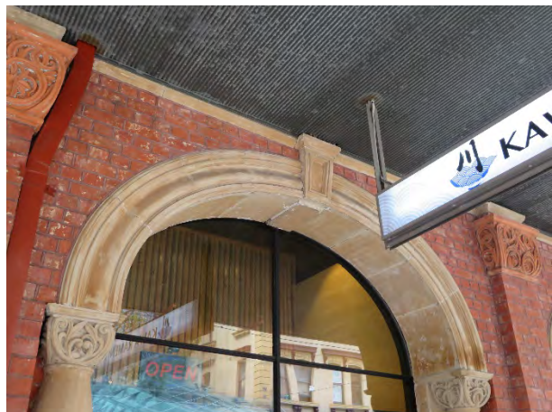
Figure 81 – Discoloured sandstone arches
