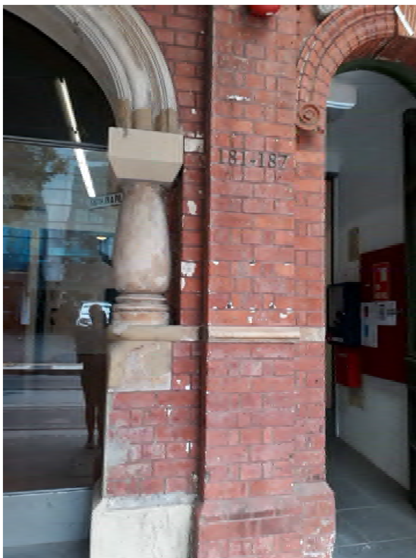
Figure 13 – Defect 15 – previous repairs to masonry
