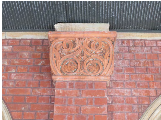
Figure 30 – Terracotta capital at ground floor on Hay Street elevation
