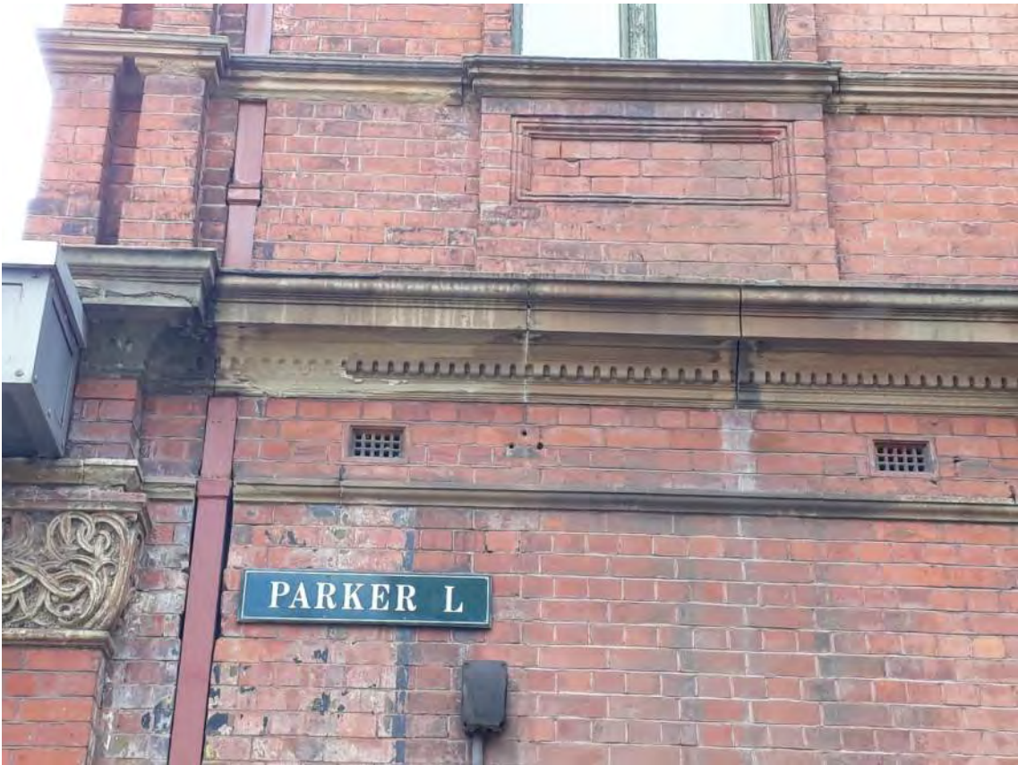
Figure 15 – Defect 17 – degraded coping stones
