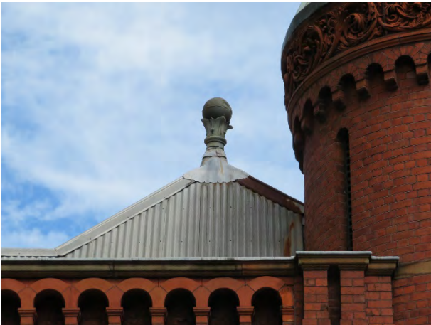
Figure 41 – Zinc finial on main ridge hipped roof
