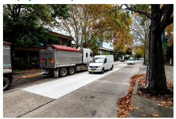
The City has been working with the Cooperative Research Centre (CRC) for Low Carbon Living to trial the use of Geopolymer, a sustainable concrete blend cement used in the production of concrete.
