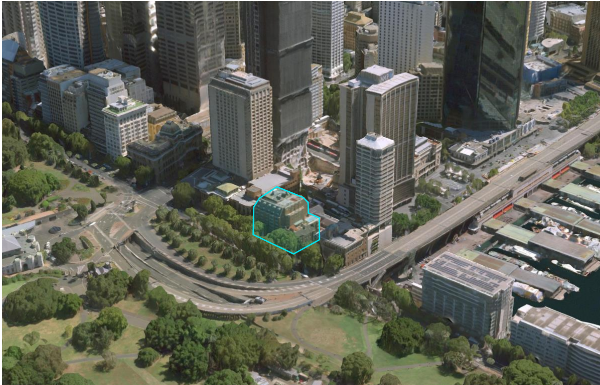
Figure 2: Photograph of the subject site in blue and surrounding area as viewed facing south west.
