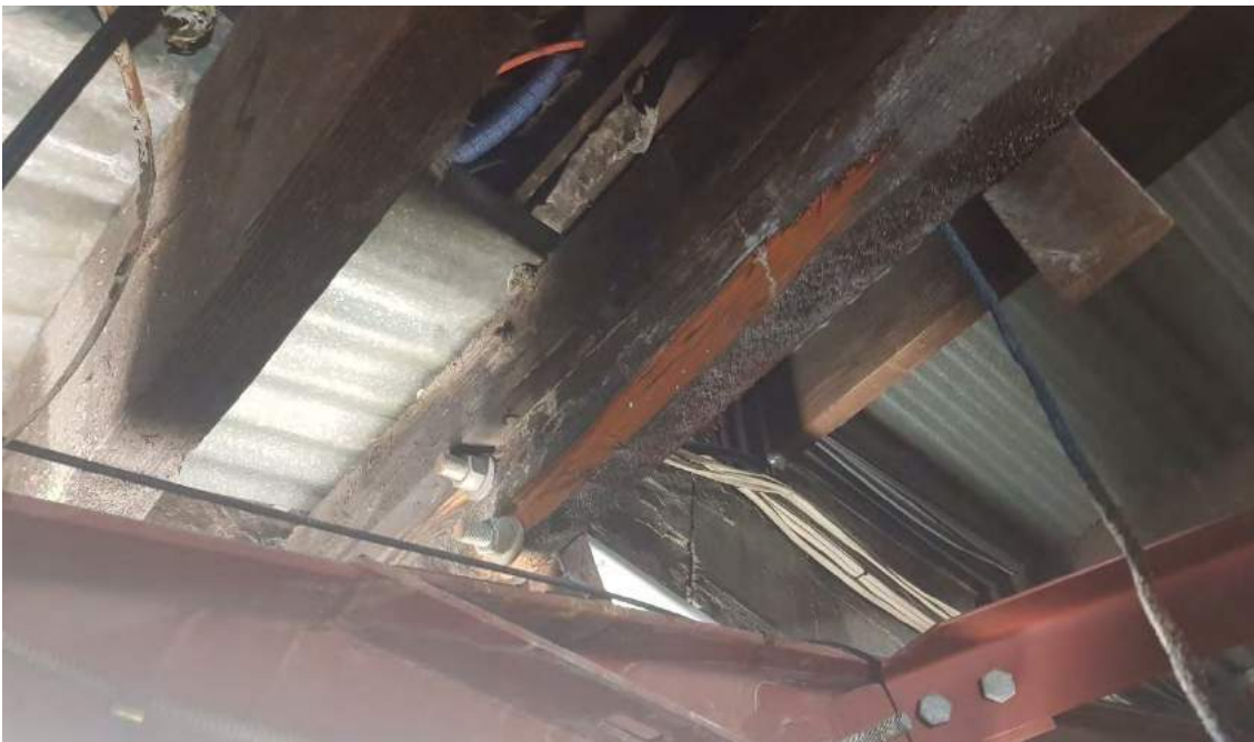
Figure 2: Original Theatre Roof – Timber Purlin Damage
