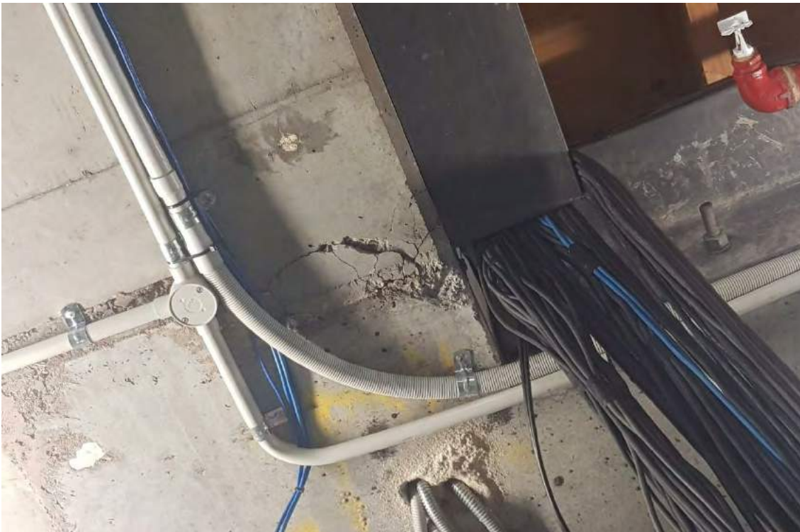
Figure 30: Minor Cracking – Underside of New Concrete Slab
