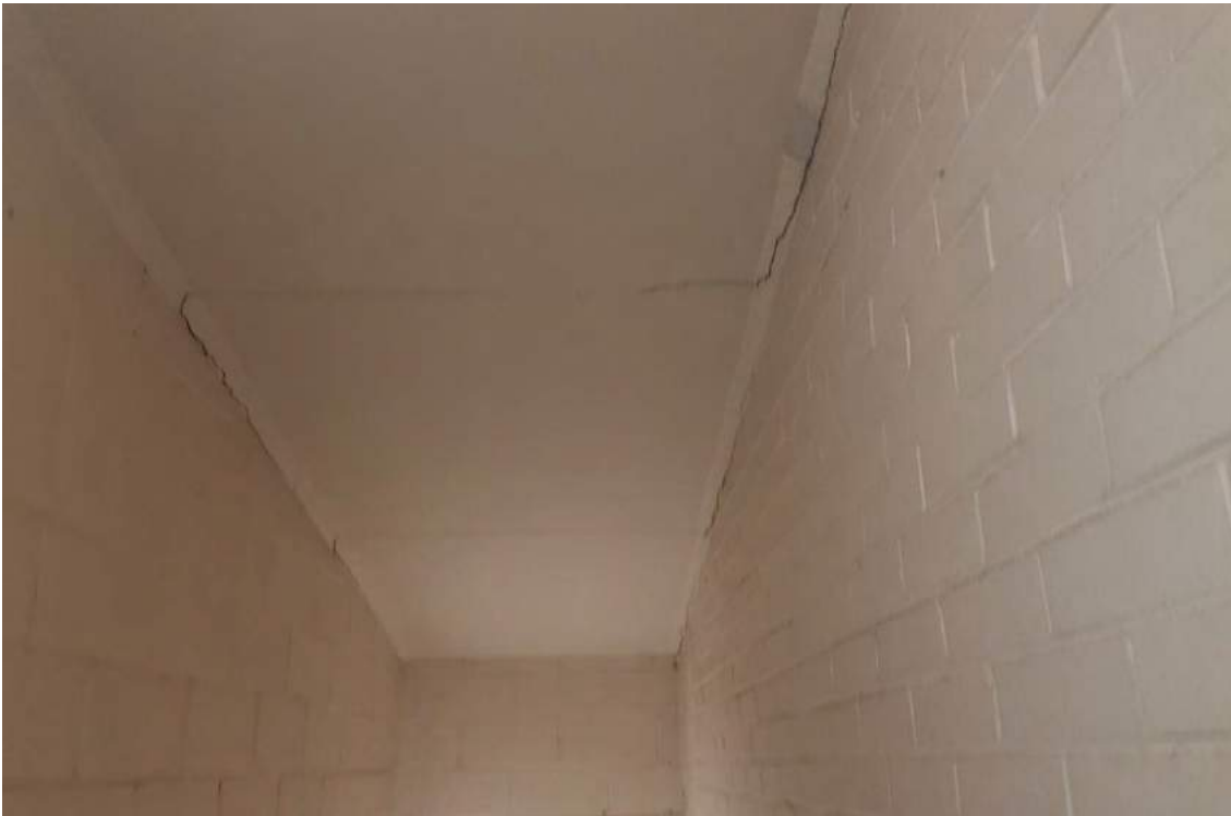
Figure 35: Minor Cracking – Stairwell Roof
