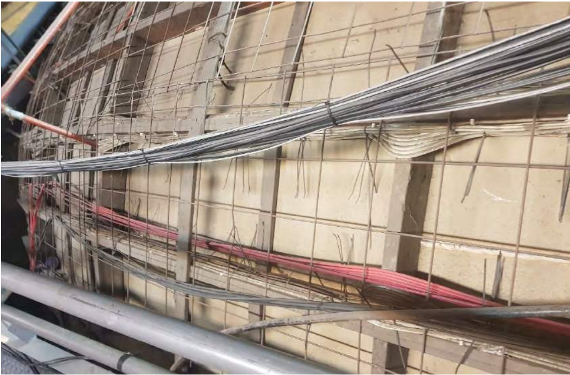
Figure 3: Original Theatre Roof – Hanging Timber Ceiling
