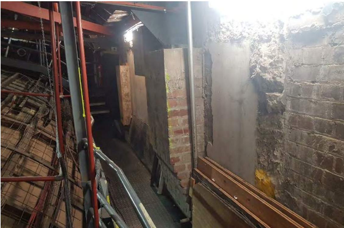
Figure 18: Original Walls – Brick Piers Supporting Roof Trusses
