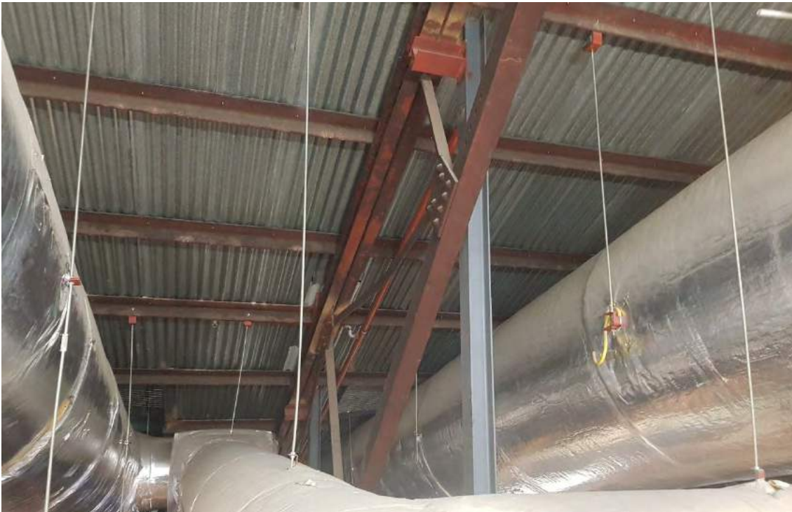
Figure 7: Original Theatre Roof – Buckled Truss Chord
