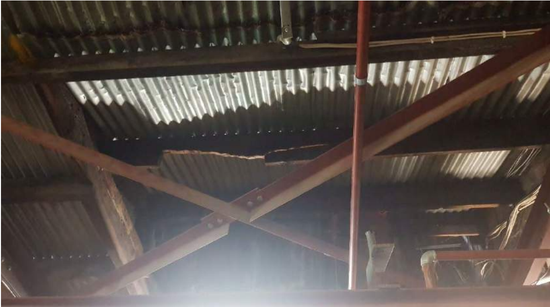
Figure 1: Original Theatre Roof – Existing Timber Purlins, Sheeting and New Steel Bracing
