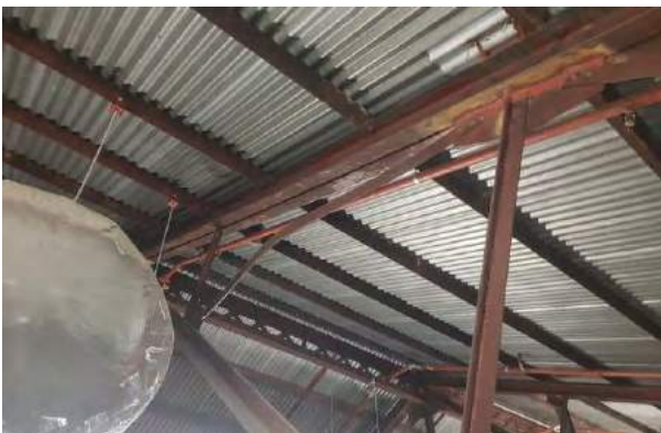
Figure 158 – Buckled truss chord in original theatre roof Source: Mott MacDonald
