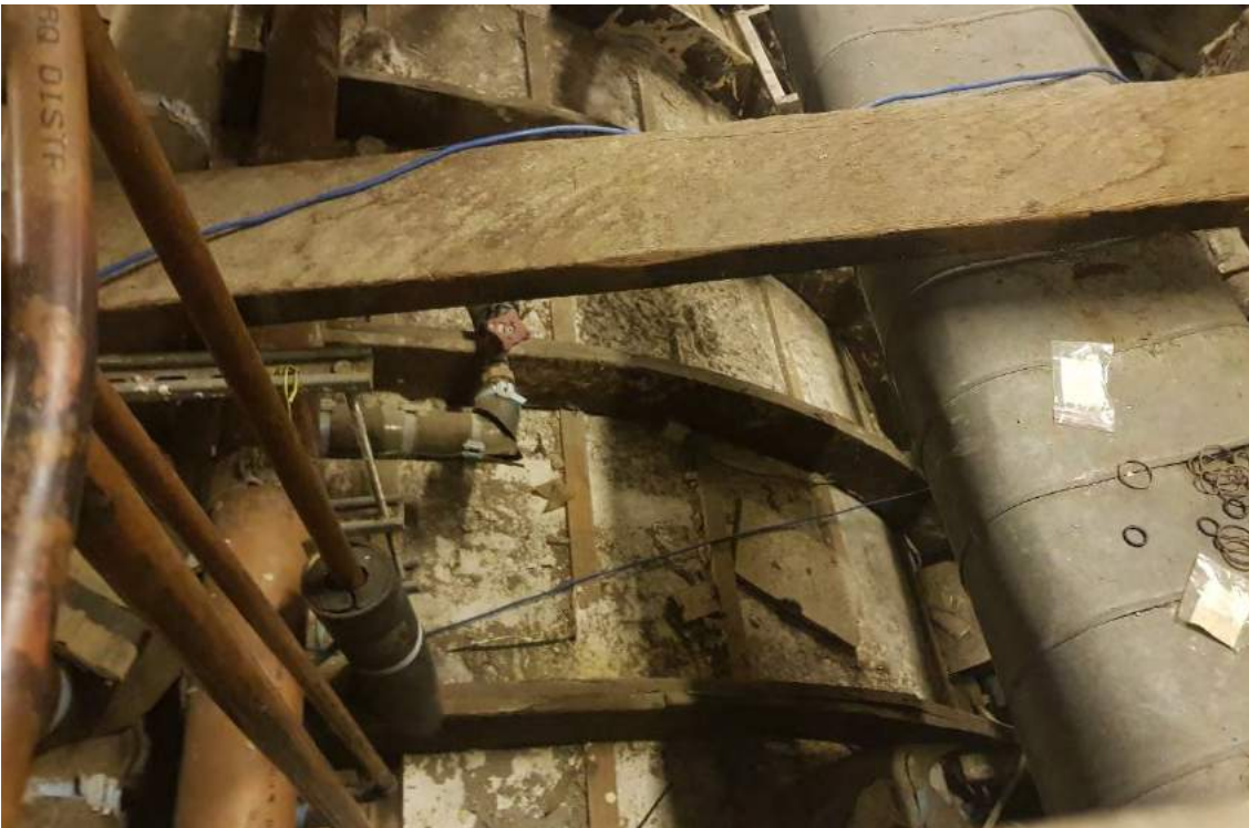
Figure 24: Dress Circle Structure – Hanging Heritage Foyer Ceiling Below
