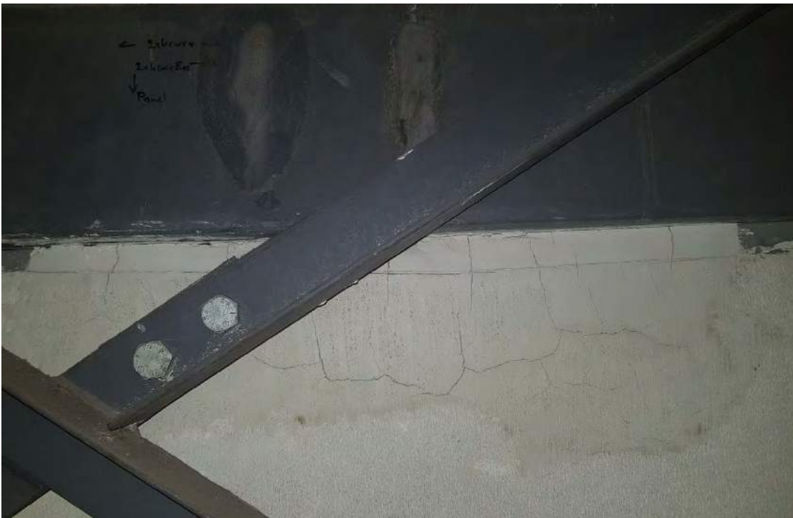
Figure 34: Minor Cracking – Crushing of Pre-Cast Panel below Steel Member
