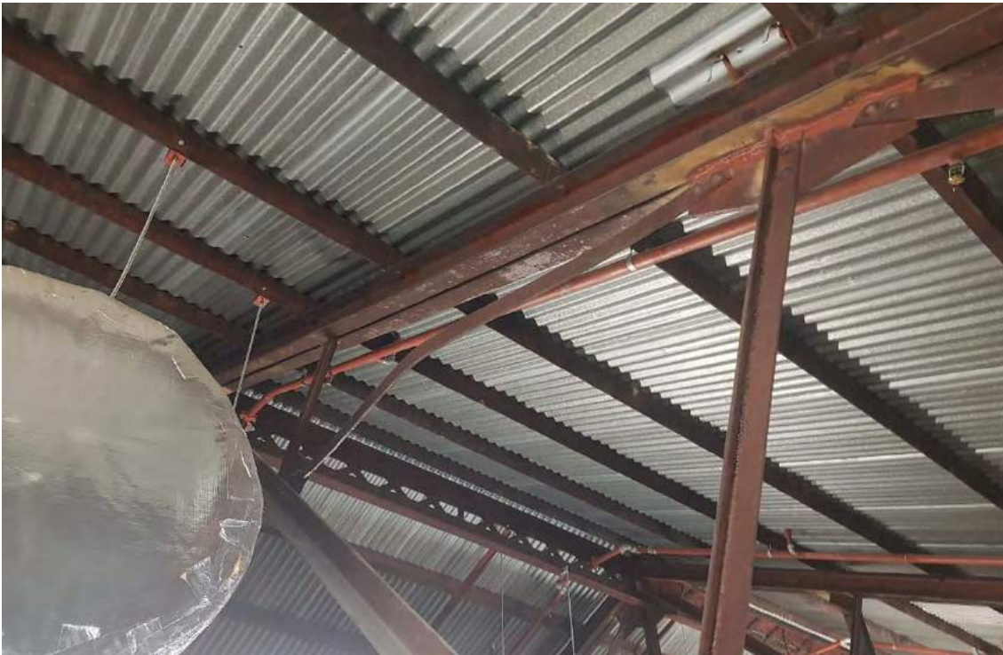
Figure 9: Original Theatre Roof – Bucked Truss Chord
