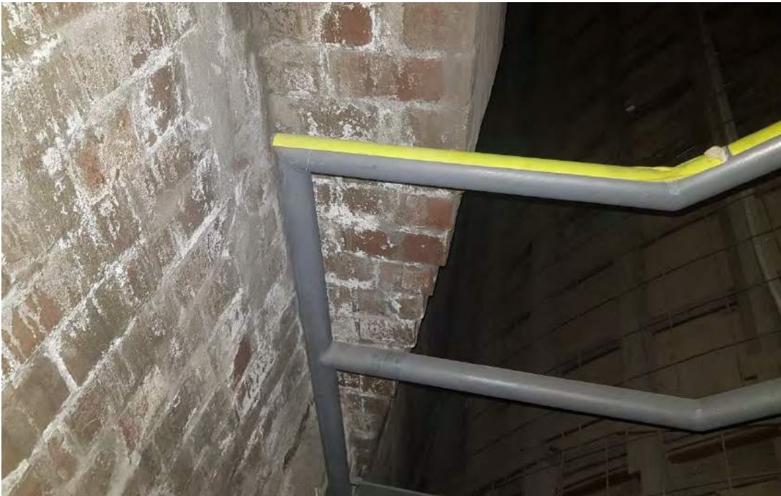
Figure 29: Roof Access Structure – Wobbly Balustrade
