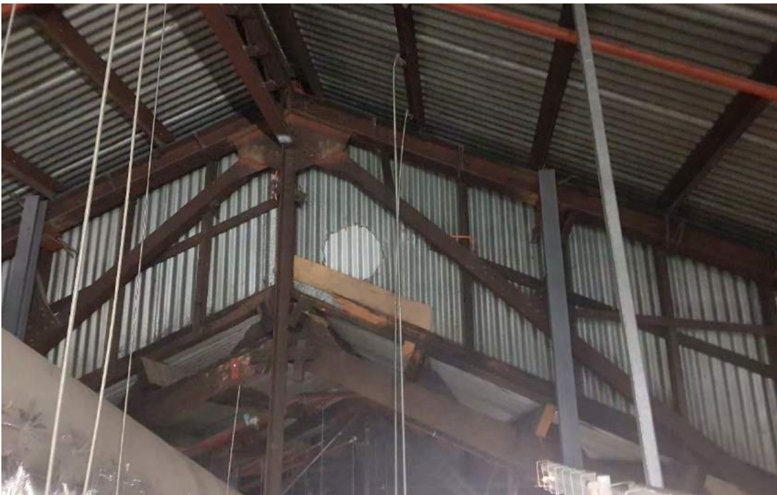
Figure 6: Original Theatre Roof – Steel Truss
