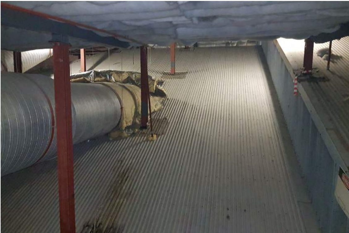
Figure 11: Original Theatre Roof – New Roof Built Above the Original Roof
