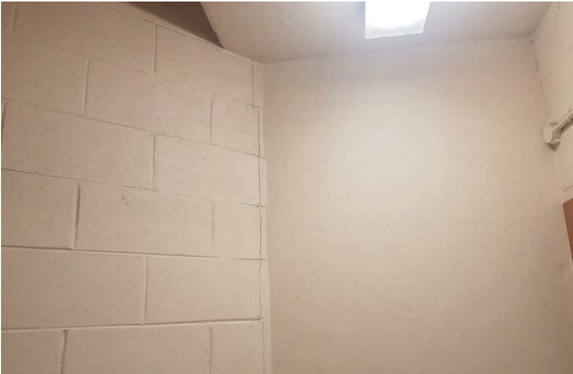
Figure 37: Minor Cracking – Stairwell Wall
