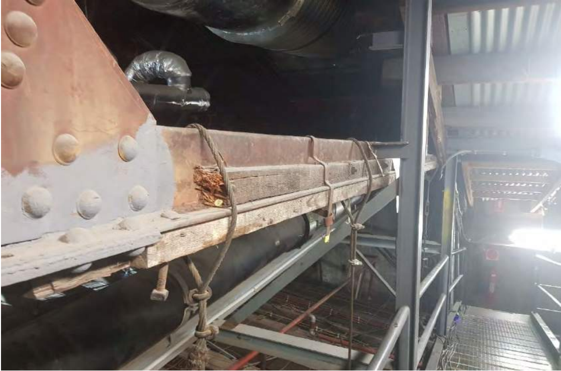
Figure 5: Original Theatre Roof – Steel Hanging Wires off Original Truss
