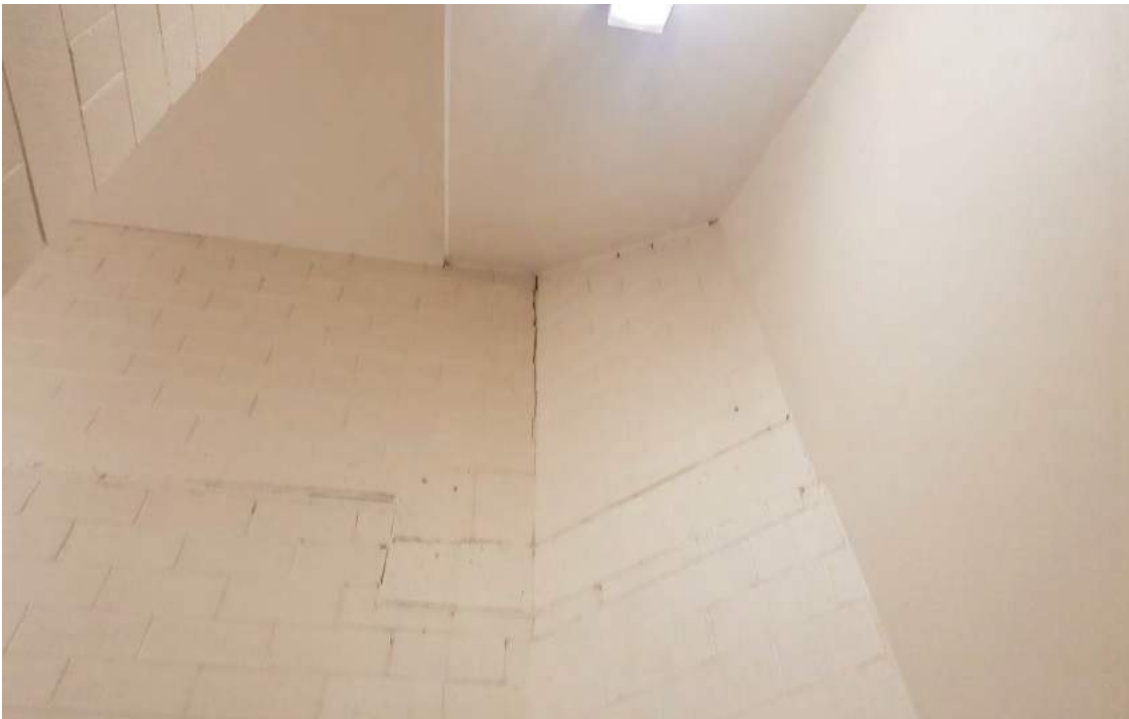
Figure 36: Minor Cracking – Stairwell Wall
