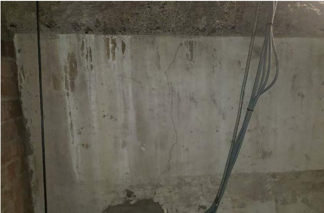
Figure 33: Minor Cracking – Cement Rendered Masonry Wall Crack
