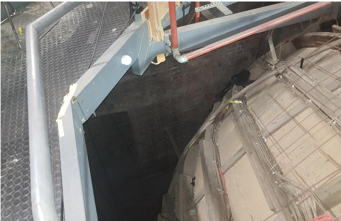
Figure 28: Roof Access Structure – Missing Bolts
