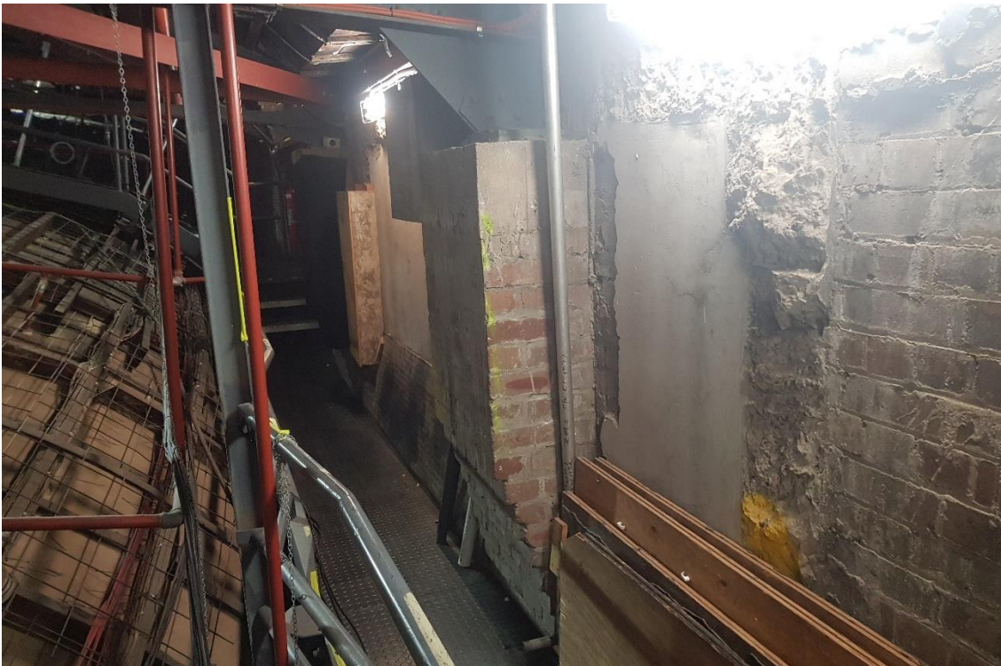
Figure 18: Original Walls – Brick Piers Supporting Roof Trusses
