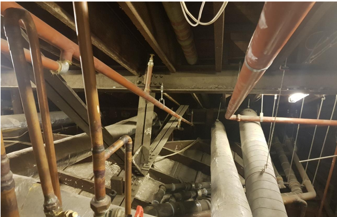
Figure 22: Dress Circle Structure - Steel Trusses and Timber Joists
