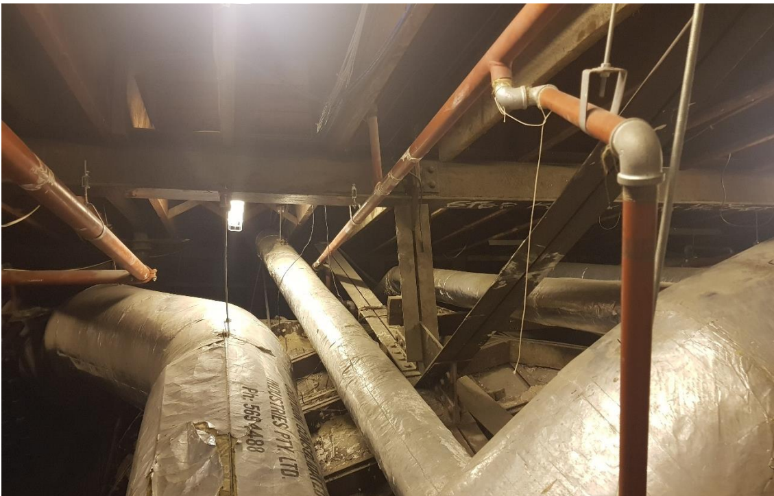
Figure 20: Dress Circle Structure – Steel Trusses and Timber Joists
