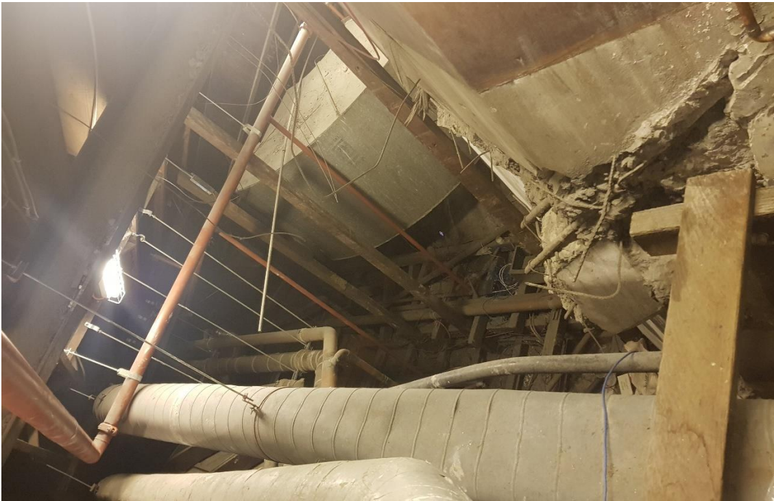
Figure 23: Dress Circle Structure – Hanging Heritage Foyer Ceiling Below
