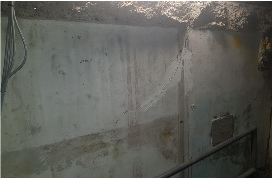
Figure 31: Minor Cracking – Diagonal Crack in the Cement Rendered Masonry Wall
