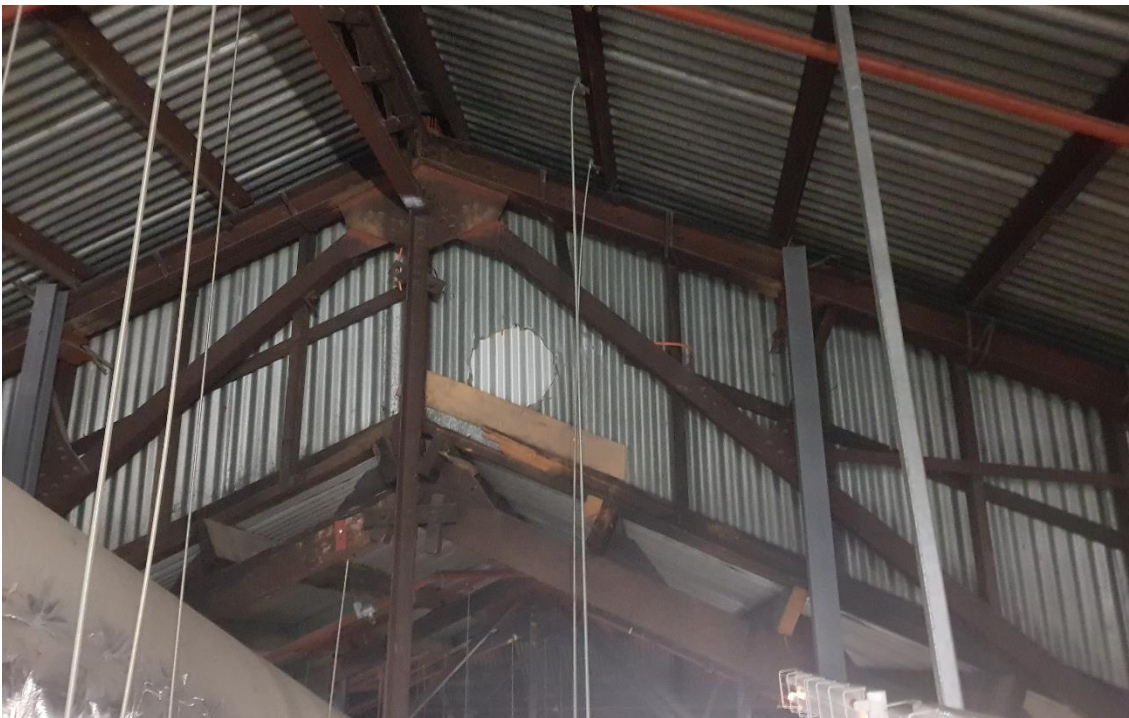
Figure 6: Original Theatre Roof – Steel Truss
