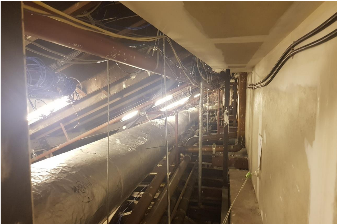
Figure 21: Dress Circle Structure - Steel Trusses and Timber Joists
