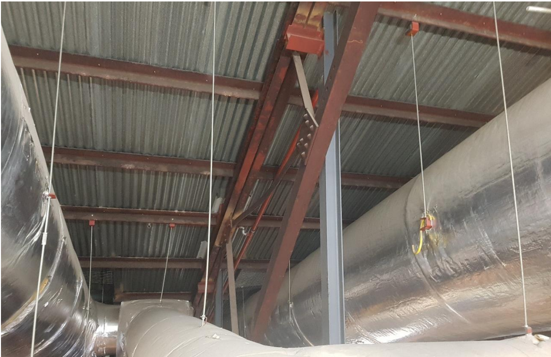
Figure 7: Original Theatre Roof – Buckled Truss Chord
