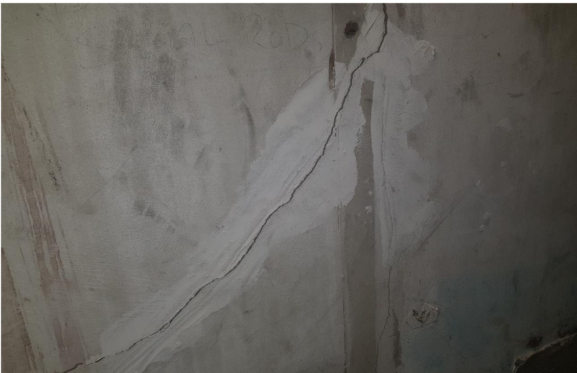
Figure 32: Minor Cracking – Close up of Cement Rendered Masonry Wall Crack
