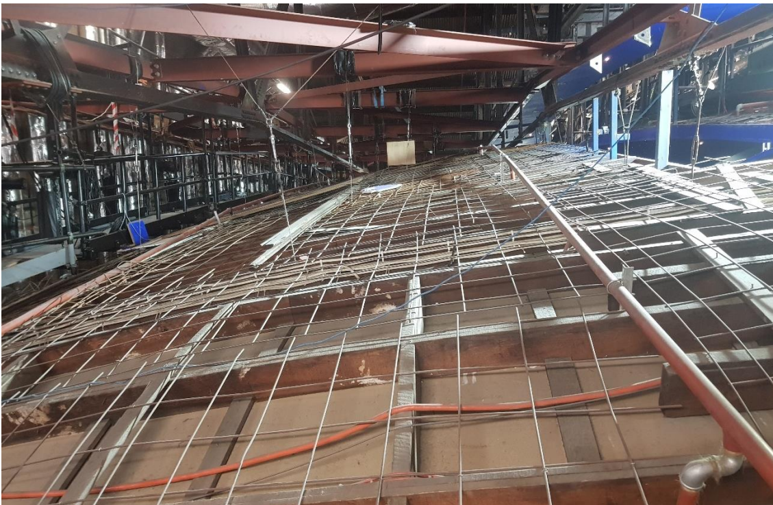
Figure 4: Original Theatre Roof – Hanging Timber Ceiling
