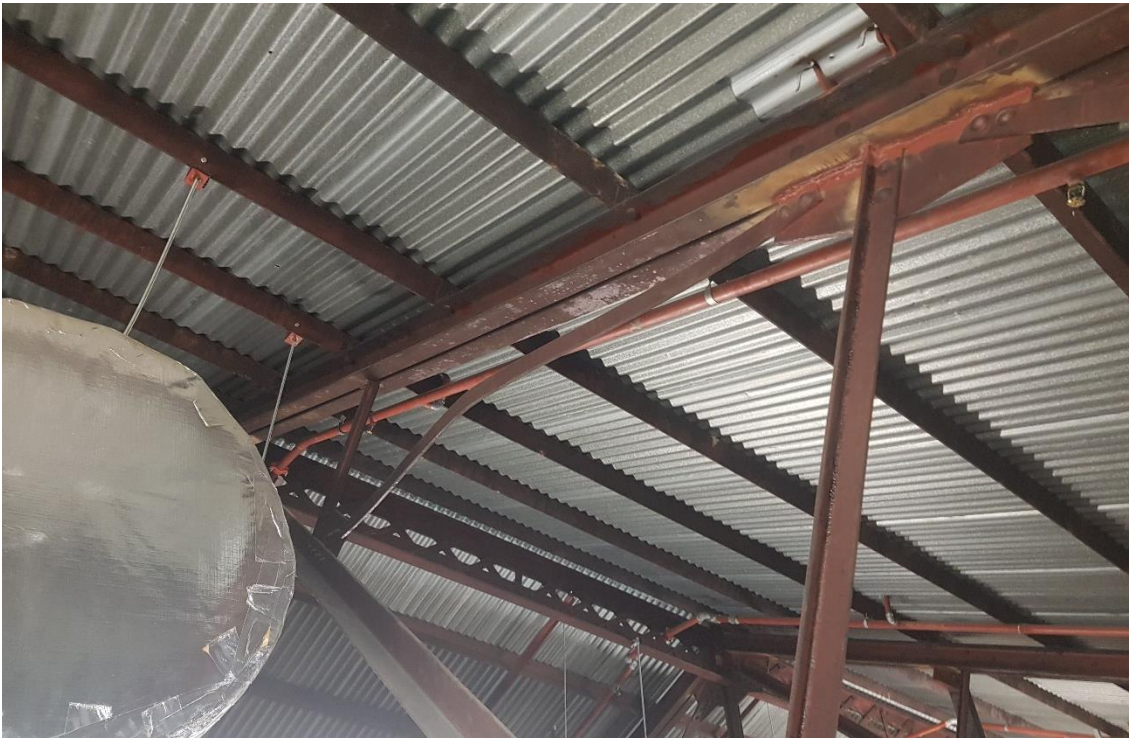
Figure 9: Original Theatre Roof – Bucked Truss Chord
