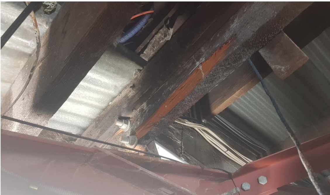
Figure 2: Original Theatre Roof – Timber Purlin Damage
