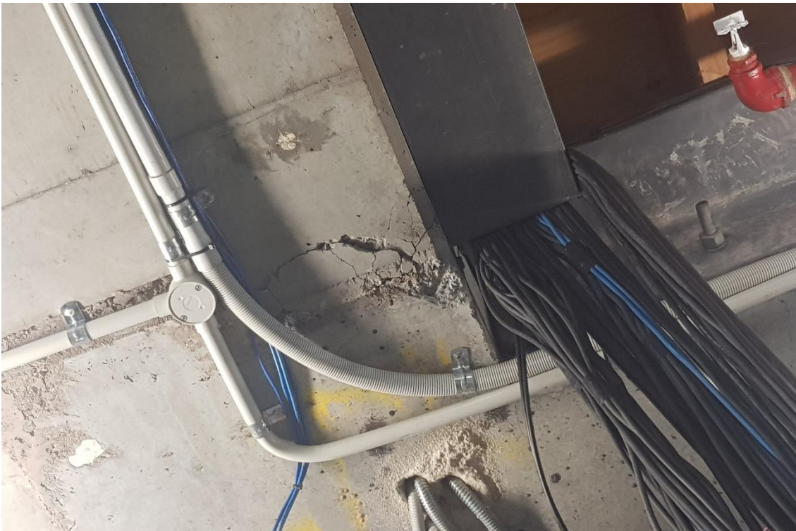
Figure 30: Minor Cracking – Underside of New Concrete Slab
