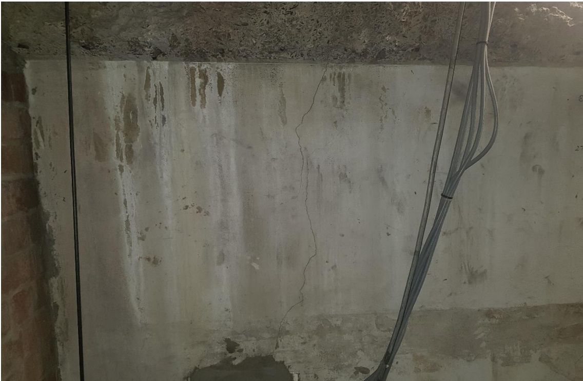
Figure 33: Minor Cracking – Cement Rendered Masonry Wall Crack
