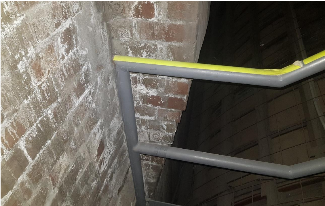
Figure 29: Roof Access Structure – Wobbly Balustrade
