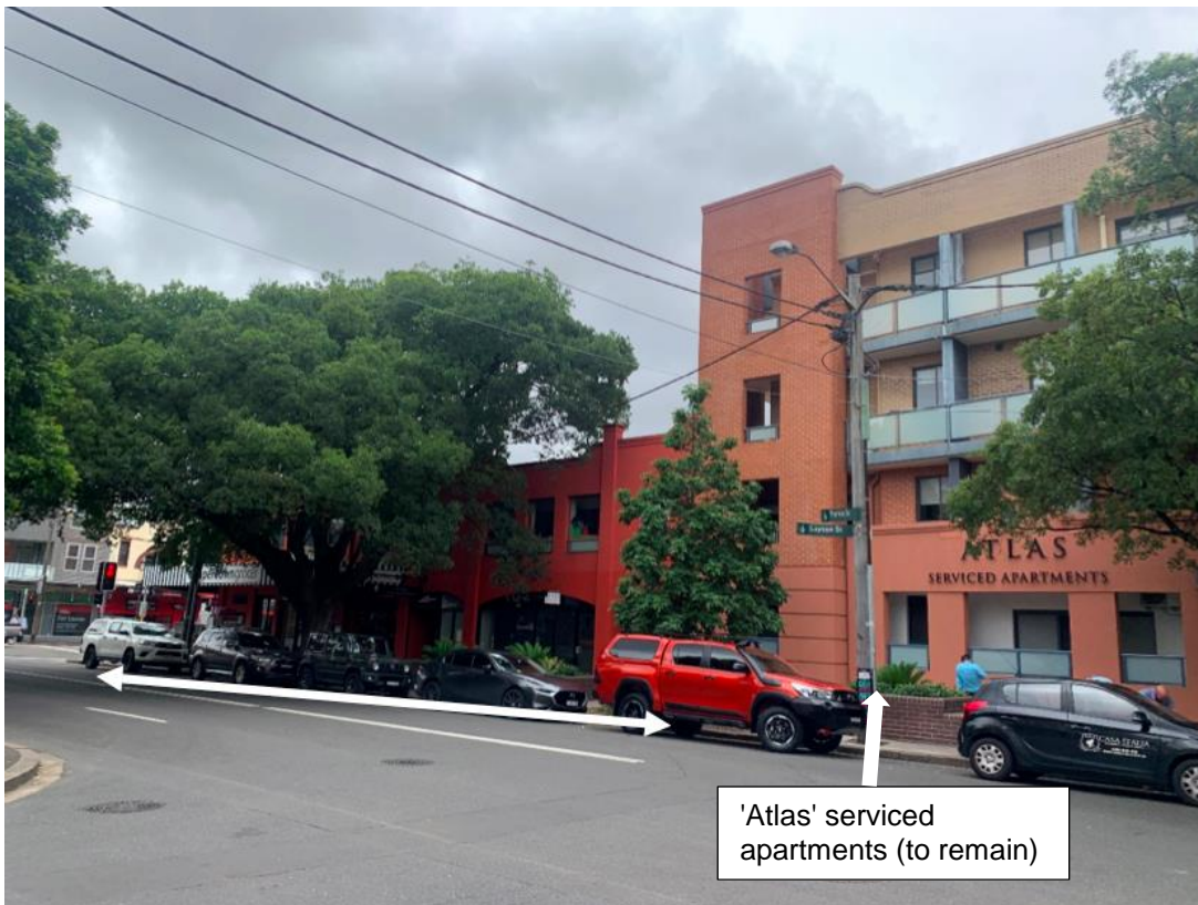
Figure 4: Site as viewed from Layton Street, with existing Camperdown Cellars building to be demolished and the Atlas Serviced Apartments to be retained
