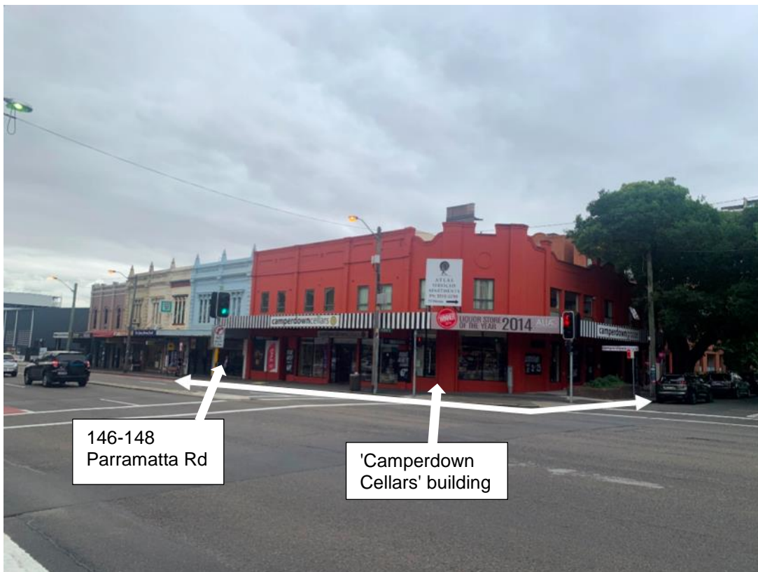
Figure 2: View from the intersection of Parramatta Road and Layton Street, with the existing buildings to be demolished
