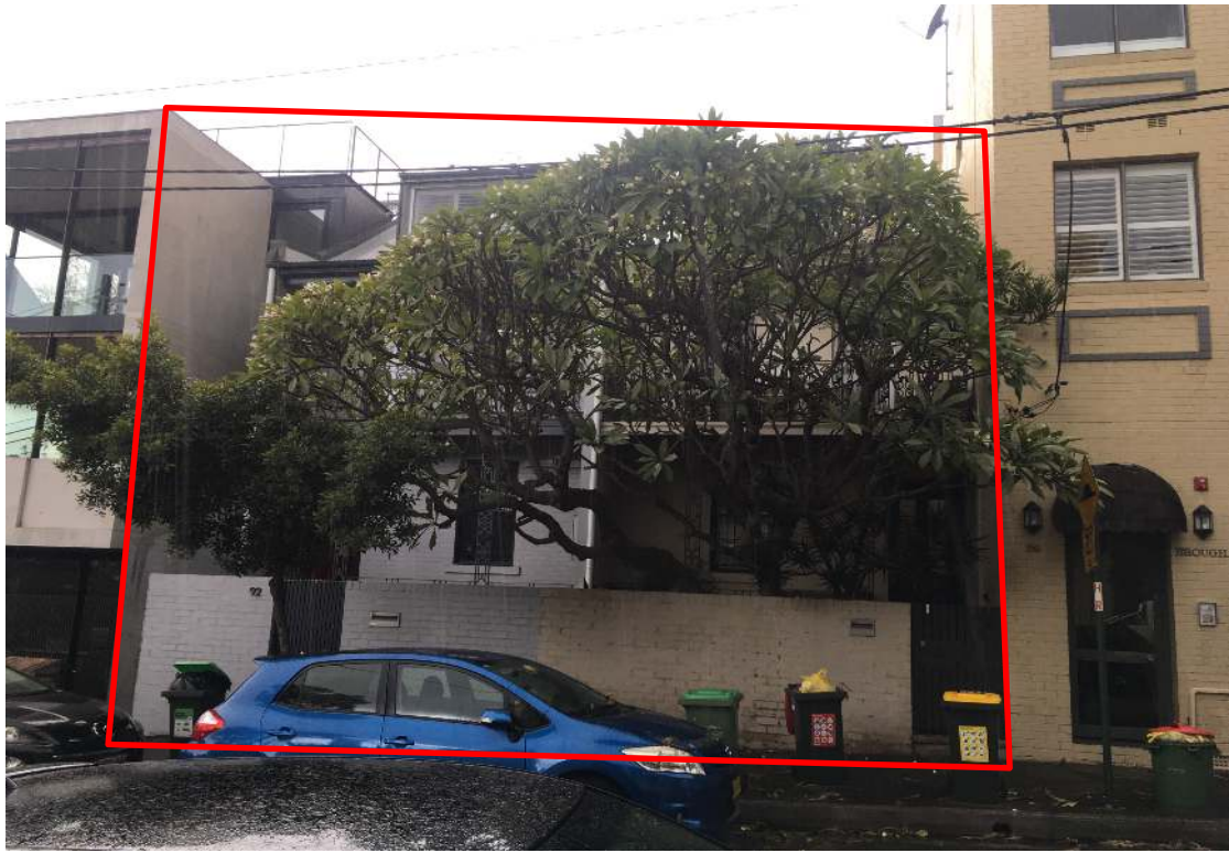
#92 (left) and #94 (right) Brougham Street
