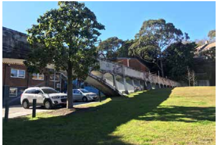
View to Johnsons Creek Aqueduct
