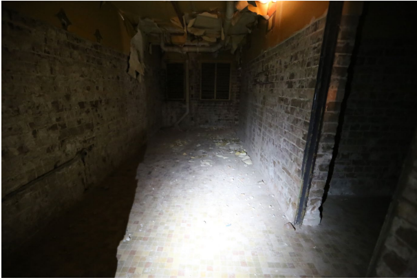
Figure 41 – Exposed brick area in the south-west corner. Including original tiled floor. Former bathrooms.
