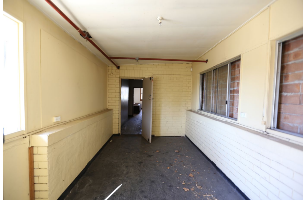
Figure 115 – View east, toward the formerly exposed western wall of level two. The doorway was originally provided access directly to the rooftop.
