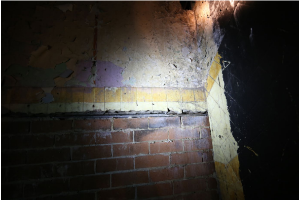
Figure 62 – Exposed brick and original tile on the western and northern walls, painted black on the northern wall.
