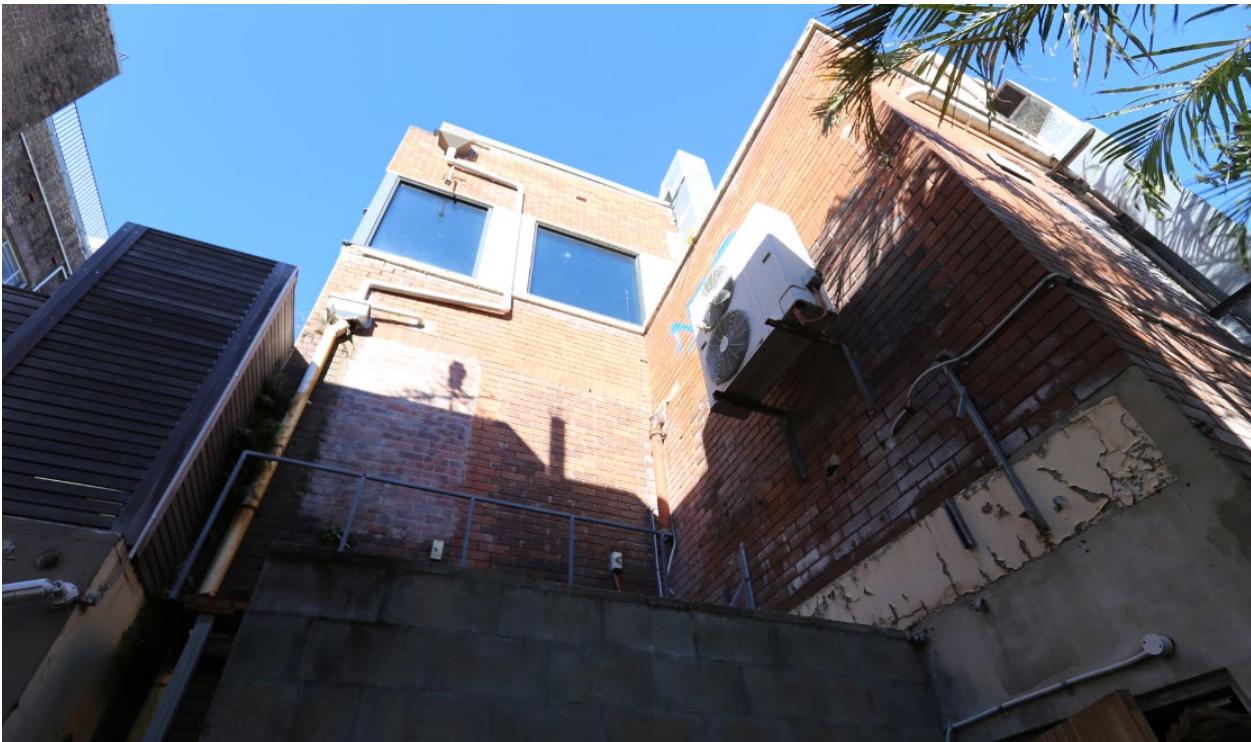
Figure 21 – View of the rear (western) façade of the subject Hotel. View from within the subject site. Note areas of infilled windows on the ground floor. Windows on the second floor were constructed in 1997 as part of the balcony infill.
