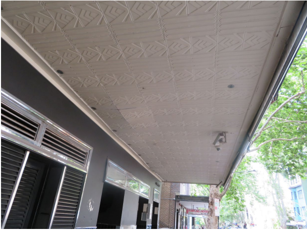
Figure 10 – Pressed metal ceiling
