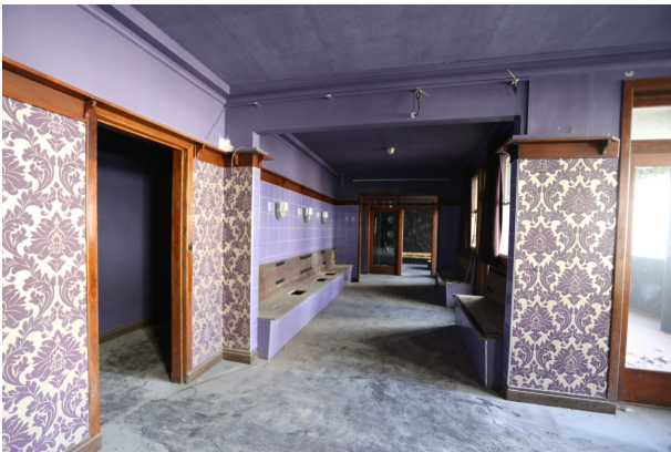
Figure 91 – View north toward the north-east corner of the first-floor. Original timber detail and cornices, contemporary wall tiles and wallpaper.
