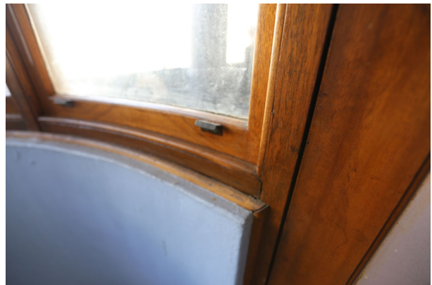
Figure 111 – Window detail with original timber frame and handles.
