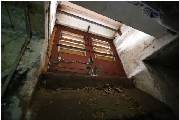
Figure 37 – Original keg shoot, located in the eastern wall in the north-east corner.
