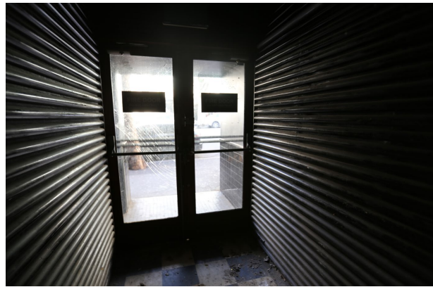
Figure 71 – Entrance doorways in original location. The doors have been upgraded for fire requirements.
