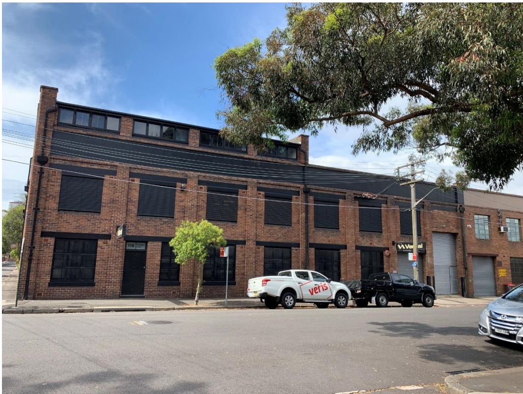
Figure 9 Non-residential commercial and industrial buildings on Wellington Street
