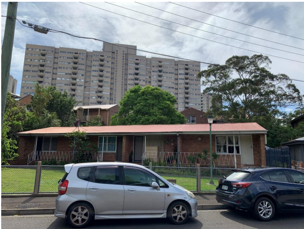
Figure 7 An example of a single-storey cottage building containing three dwellings (note the building in the background is not part of Waterloo Estate (South) stage)
