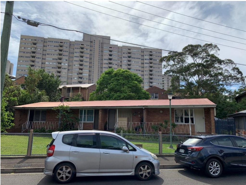
Figure 7 An example of a single-storey cottage building containing three dwellings (note the building in the background is not part of Waterloo Estate (South) stage)
