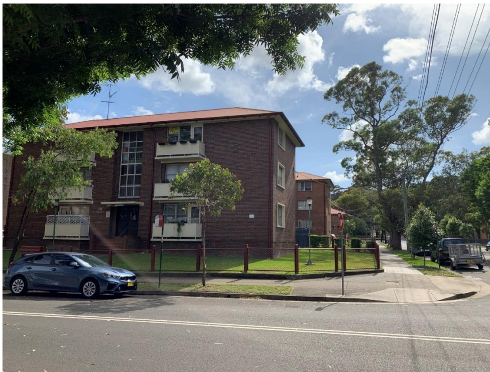
Figure 4 An example of three storey walk-up buildings (existing social housing)
