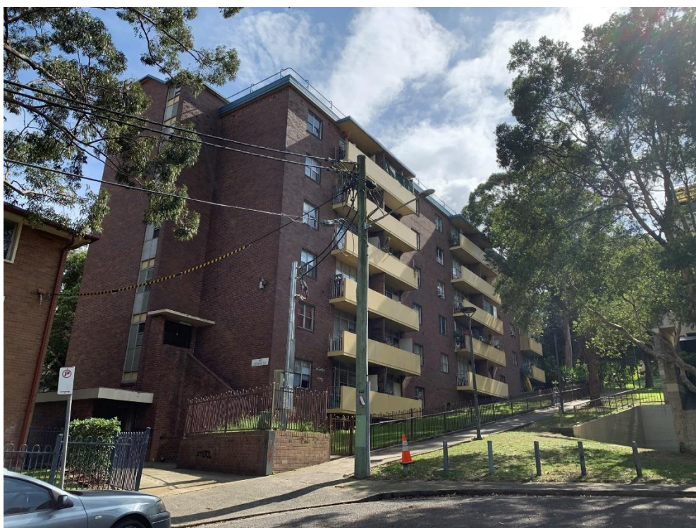
Figure 5 An example of a mid-rise building (existing social housing)
