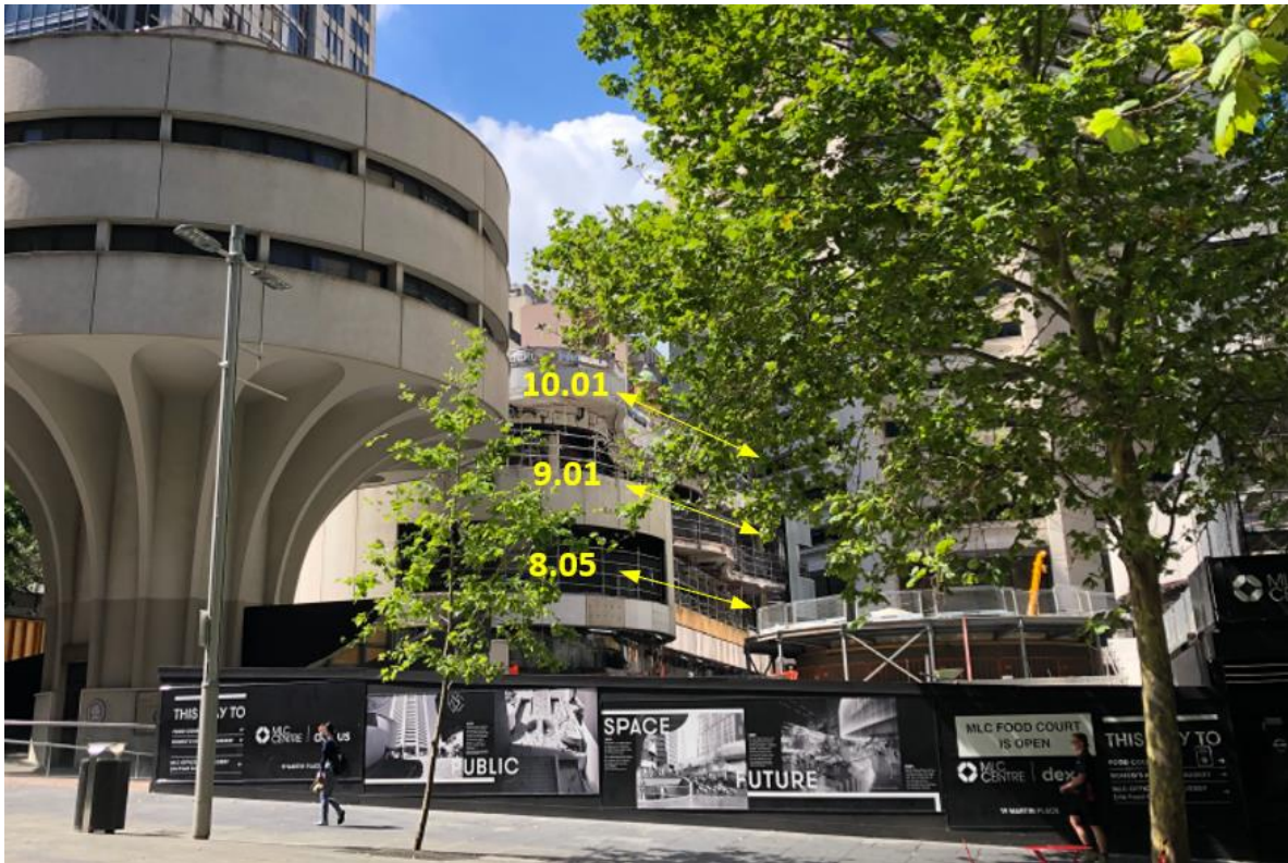
Figure 3: Site viewed from Martin Place, with tenancy locations highlighted
