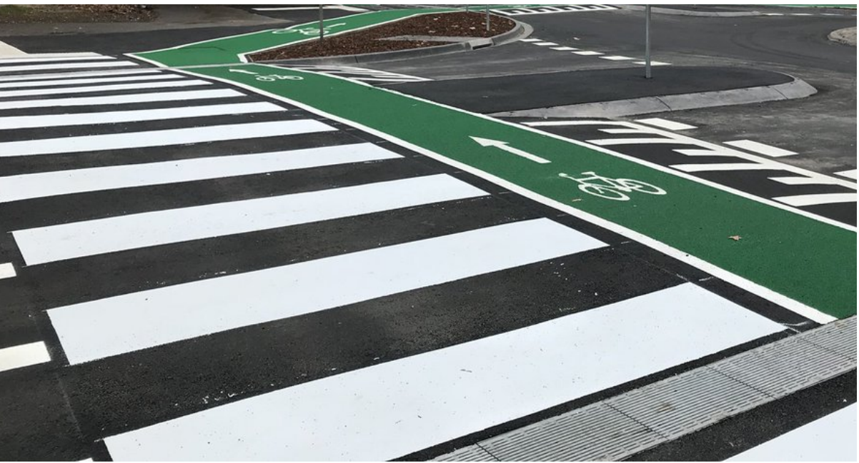
PV5 - RAISED THRESHOLD PEDESTRIAN ZEBRA CROSSING. ASPHALT AND PAINTED LINEMARKING
