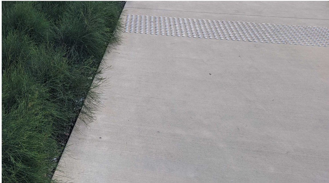
PV2 - INSITU GREEN CONCRETE PAVEMENT
