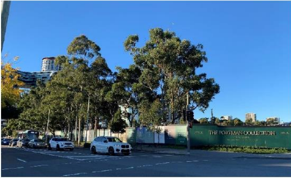
The site as viewed from Botany Road (south-west)
