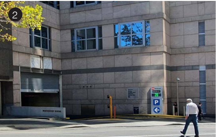
The only vehicular entry for the site is located mid block on the eastern boundary next to the Australian Club site. The existing clearance is 3.6m and is currently non-compliant .
