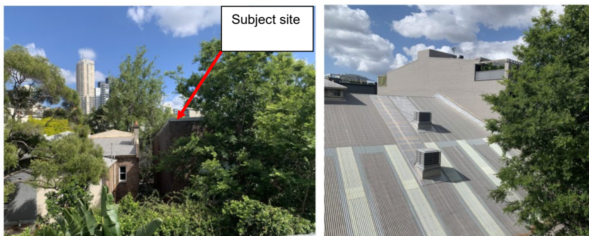
Figure 5: Residential interface with the site. (L-R) 2 storey terraces on Barcom Ave to south-east of site, taken from balcony of 9/61-63 McLachlan Ave (fourth floor) and view towards four storey apartment building at 61-63 McLachlan Ave to south of site (photograph taken from inside existing building on subject site (rear, second floor))
